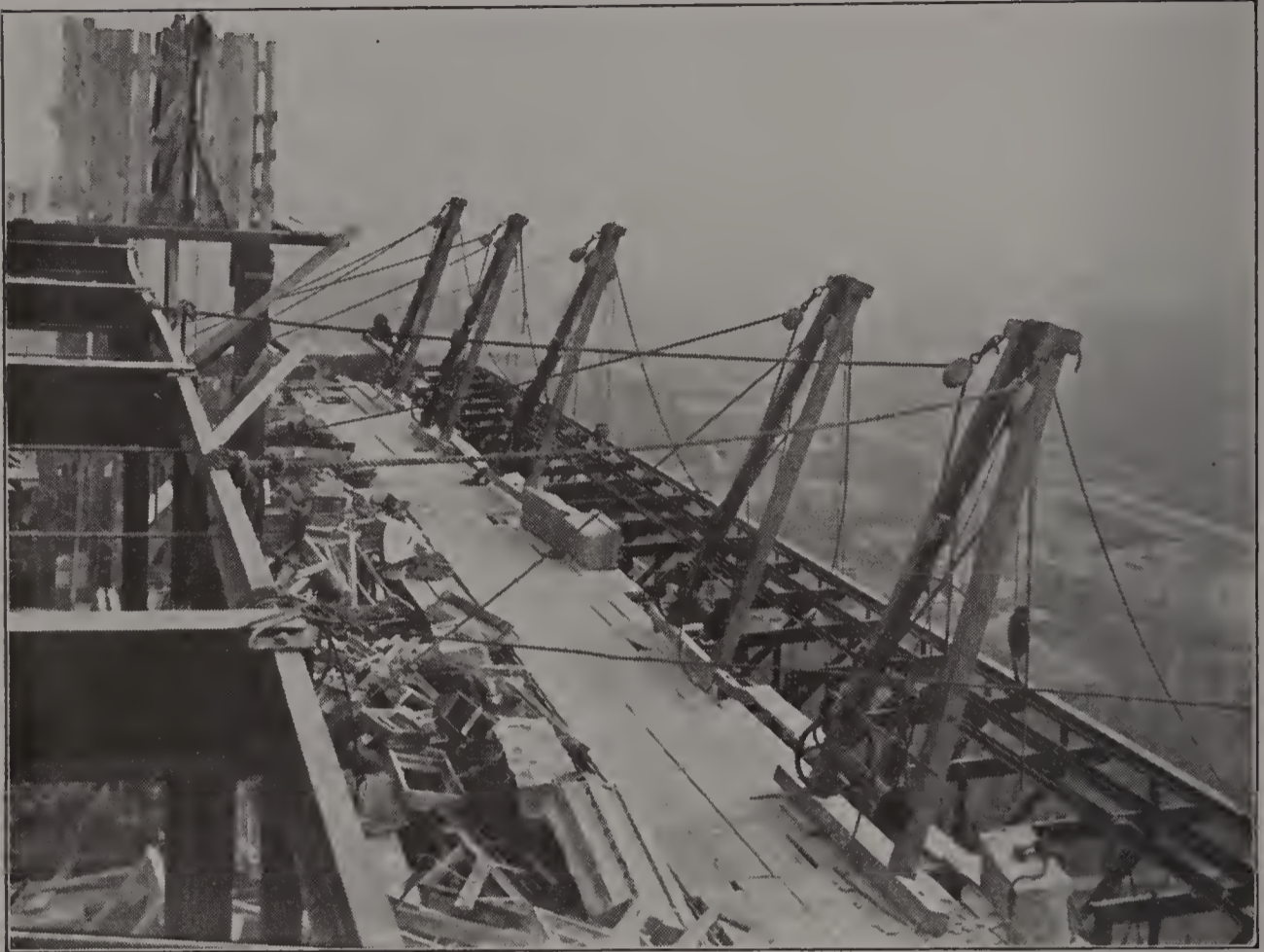
FIG. 28. A ROW OF BREAST DERRICKS USED FOR SETTING STONE.
