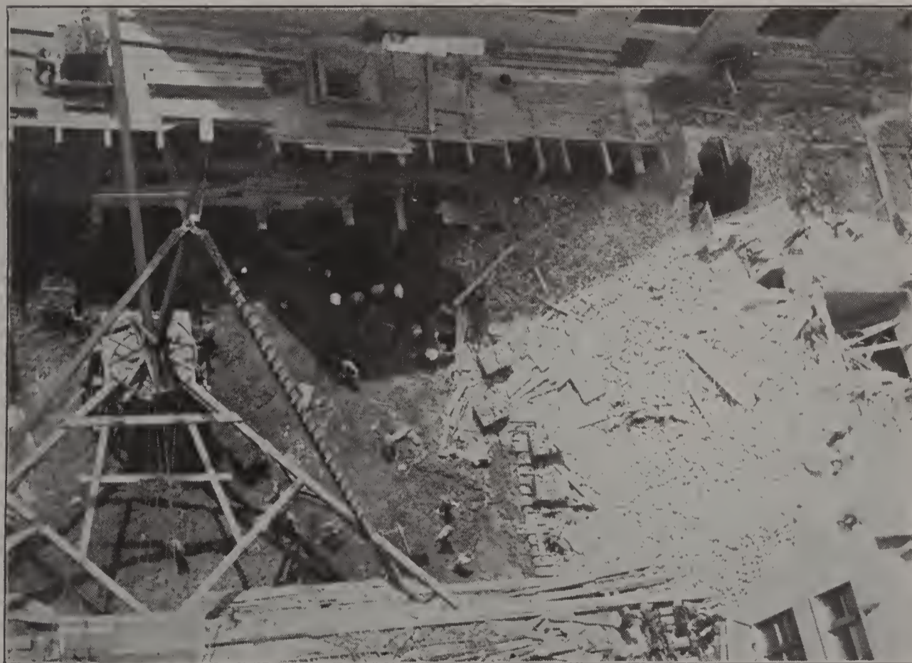
FIG. 5. EXCAVATING FOR A LARGE OFFICE BUILDING.
