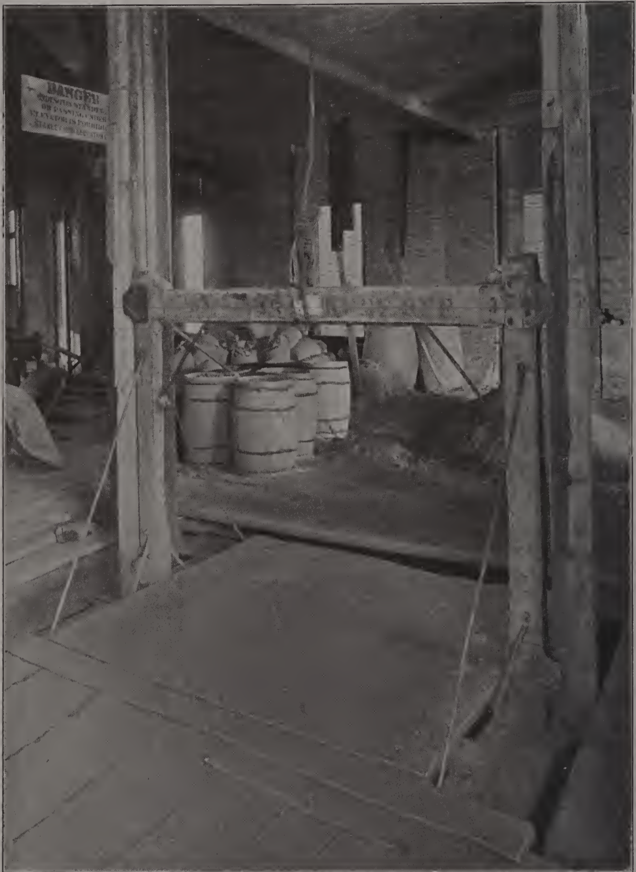
FIG. 15. AN UNPROTECTED MATERIAL HOIST AND SHAFTWAY. (The floor openings at the sides of the hoist should be covered over, and the shaftway and hoist should be guarded as indicated in paragraph 26.)
