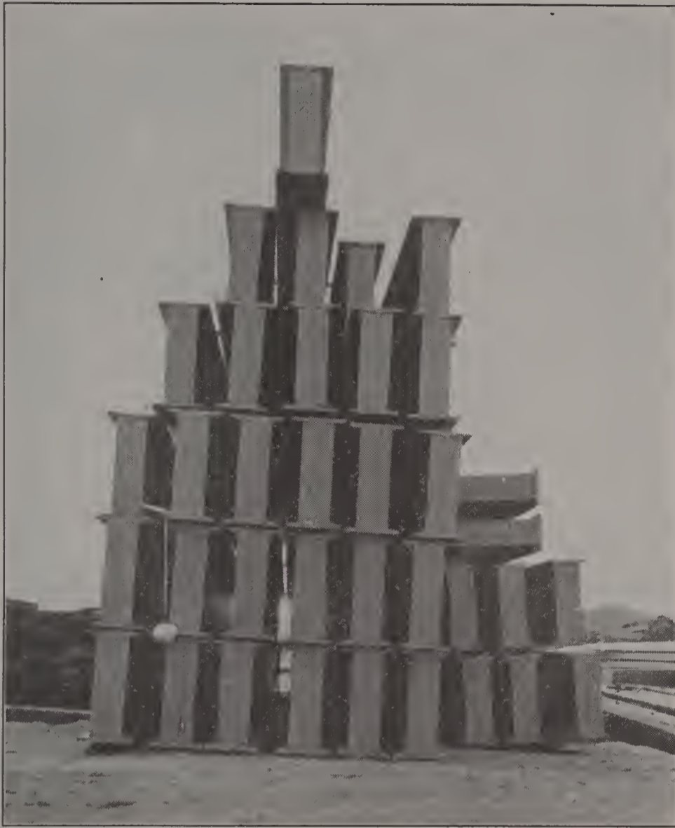
FIG. 8. UNSAFE PILING OF HEAVY STEEL GIRDERS.
