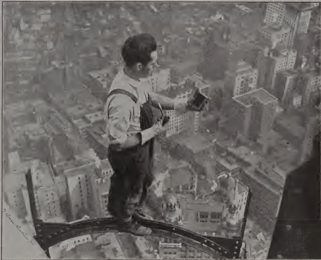
FIG. 35. A WORKMAN TAKING UNNECESSARY CHANCES.
