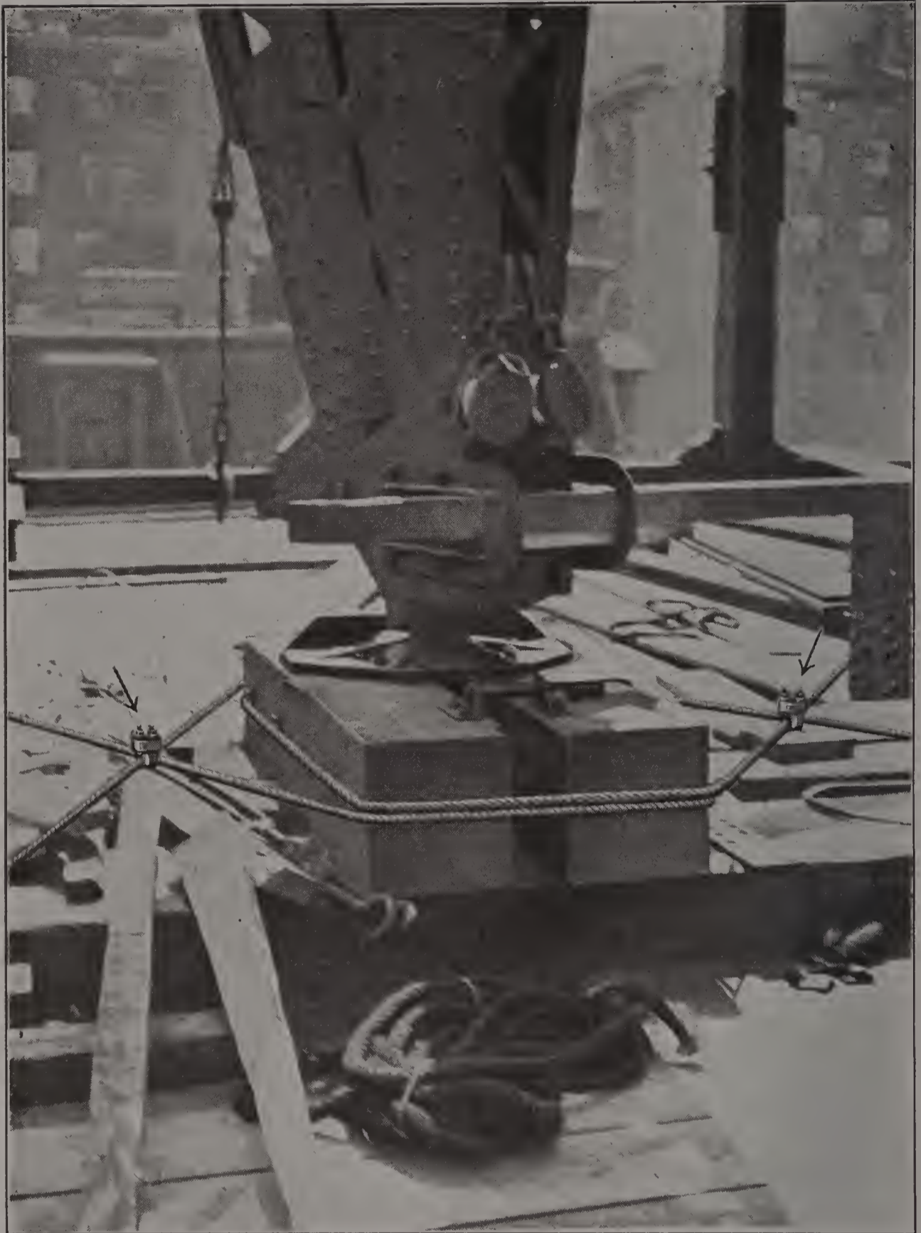
FIG. 25. AN APPROVED METHOD FOR ANCHORING DERRICK FOOT-BLOCKS.
