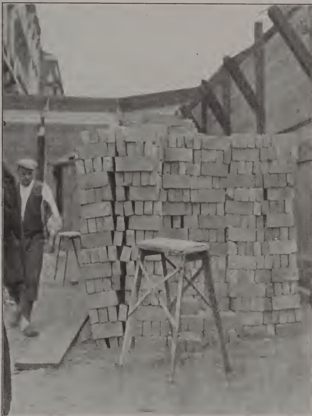
FIG. 48. A DANGEROUS PILE OF BRICKS.
