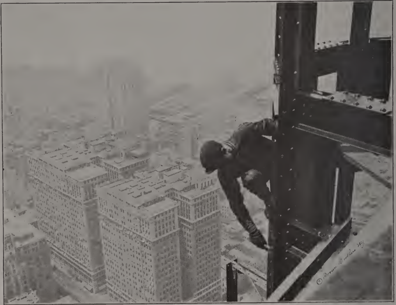
FIG. 45. PAINTING THE STEELWORK OF A "SKYSCRAPER".
