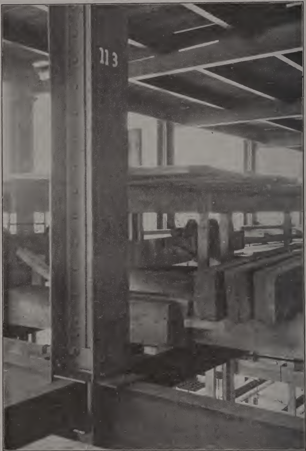
FIG. 18. PROTECTIVE COVERING FOR THE OVERHEAD-WORK OF A MATERIAL HOIST.
