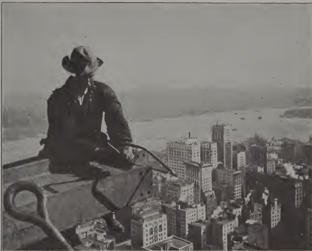
FIG. 44. WORKING UNDER DANGEROUS CONDITIONS.
