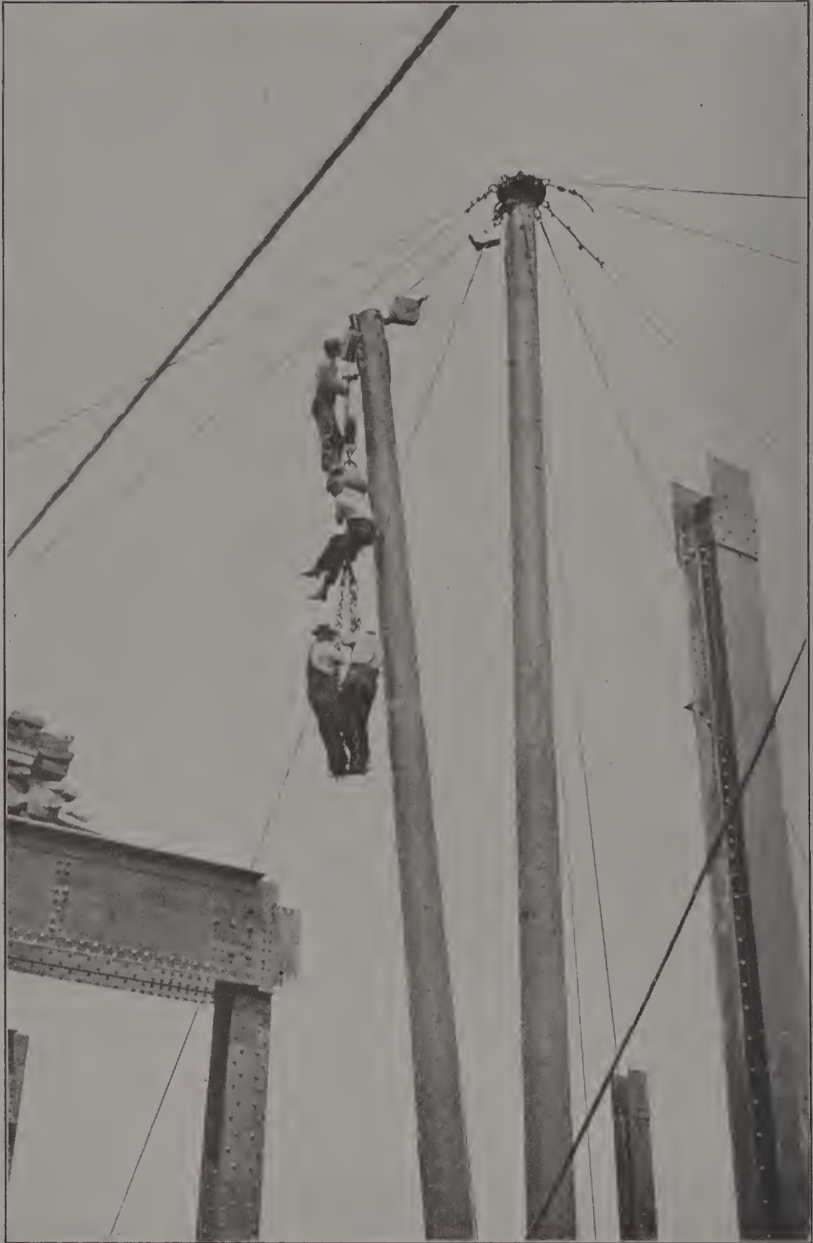
FIG. 36. STEEL MEN BEING LIFTED TO THEIR WORK.
