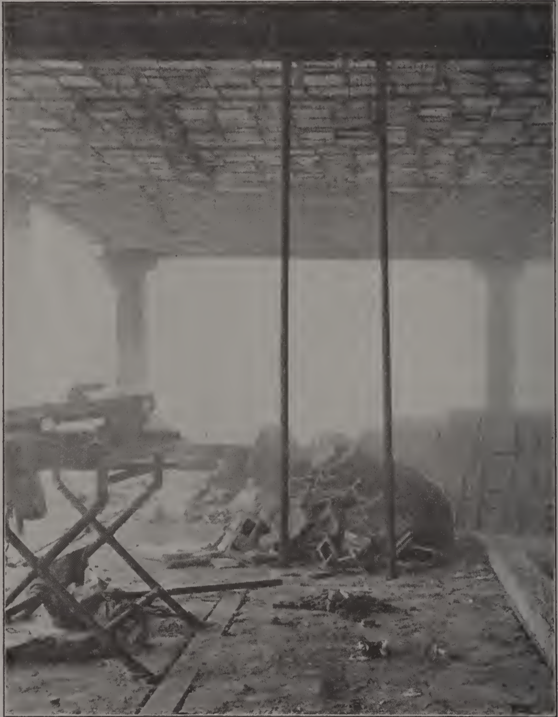
FIG. 10. THE SIGNAL CORDS ARE HERE INCLOSED IN IRON PIPES.
