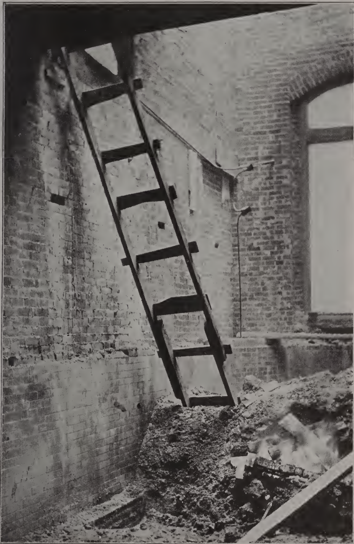
FIG. 32. A POORLY-CONSTRUCTED LADDER.
