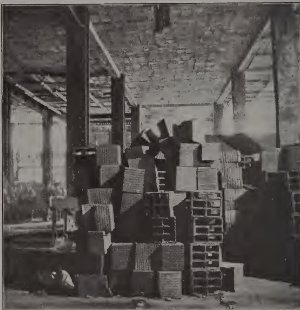
FIG. 47. POORLY-PILED FLOOR TILES.
