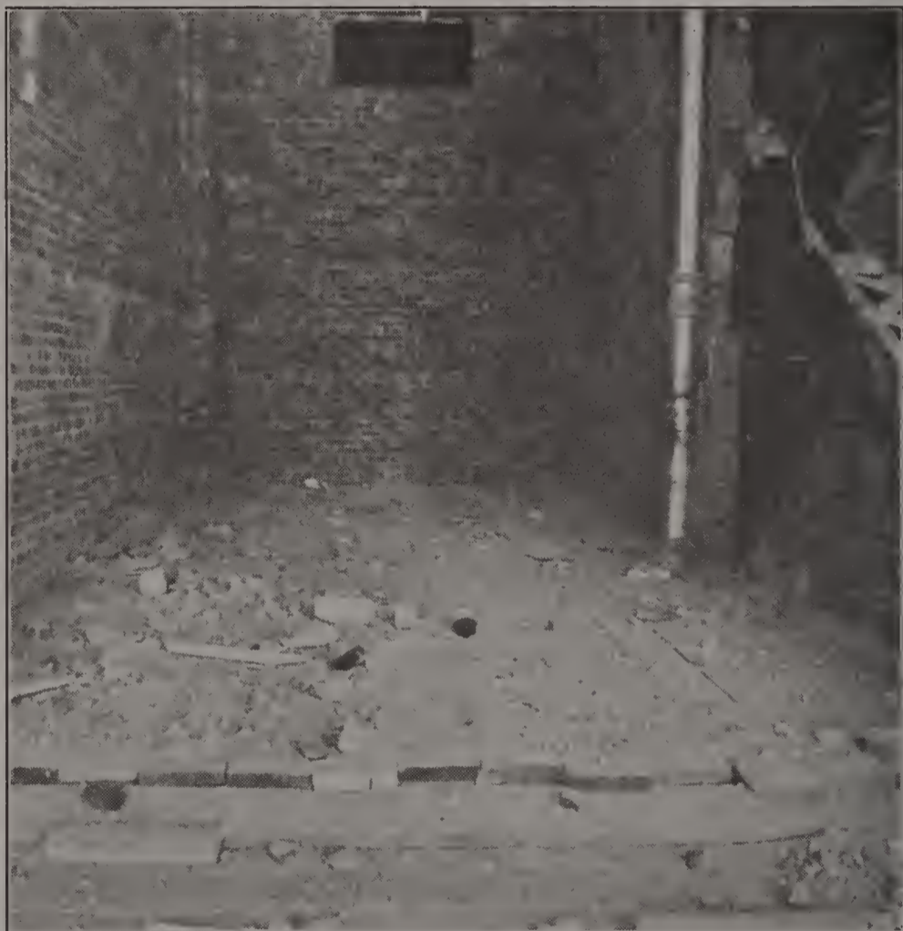
FIG. 37. PROTECTIVE PLANK FLOORING IN A VENTILATING SHAFT.
