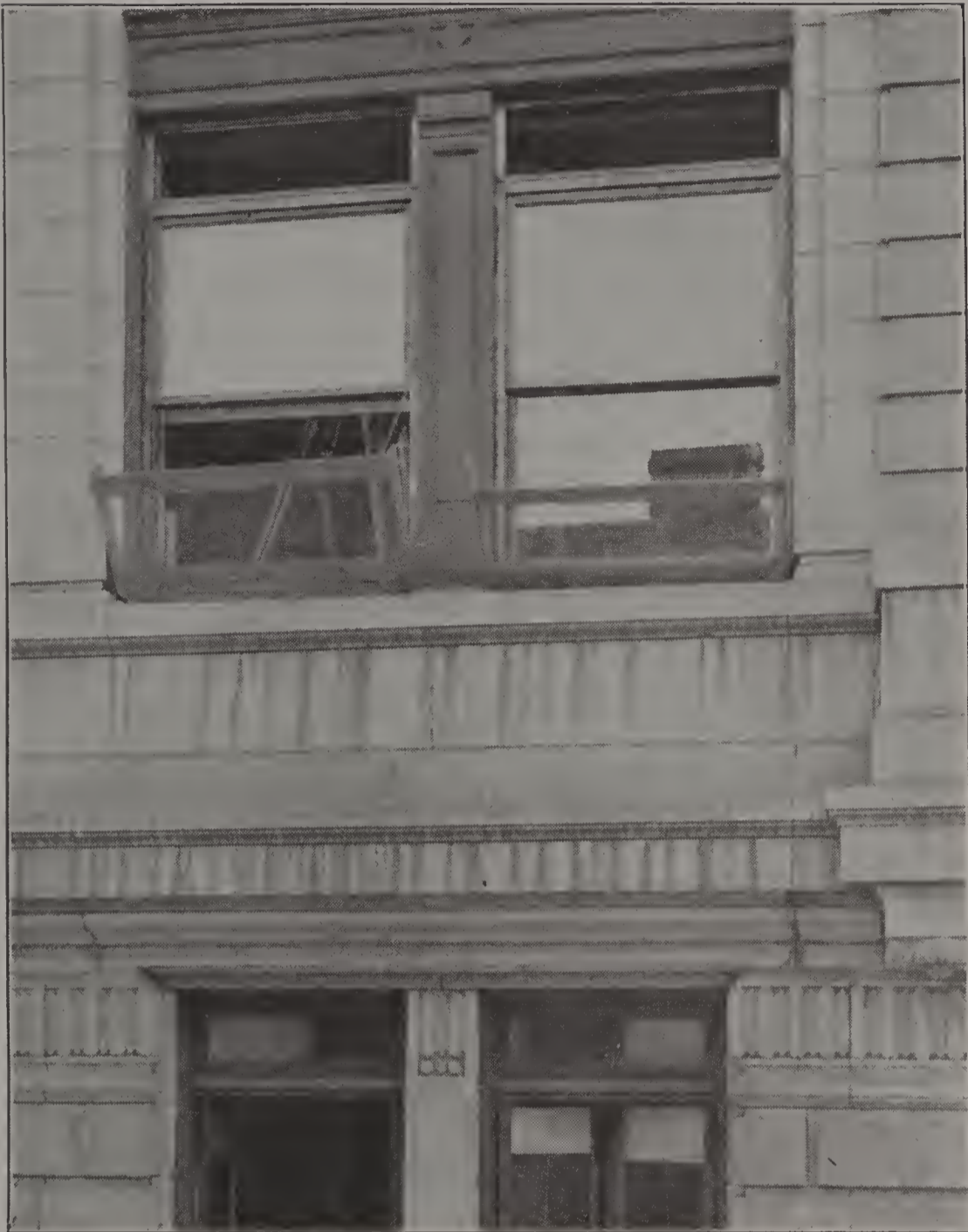
FIG. 6. A GUARD TO INTERCEPT FALLING TOOLS AND OTHER OBJECTS, WHEN MEN ARE WORKING ABOUT WINDOWS.
