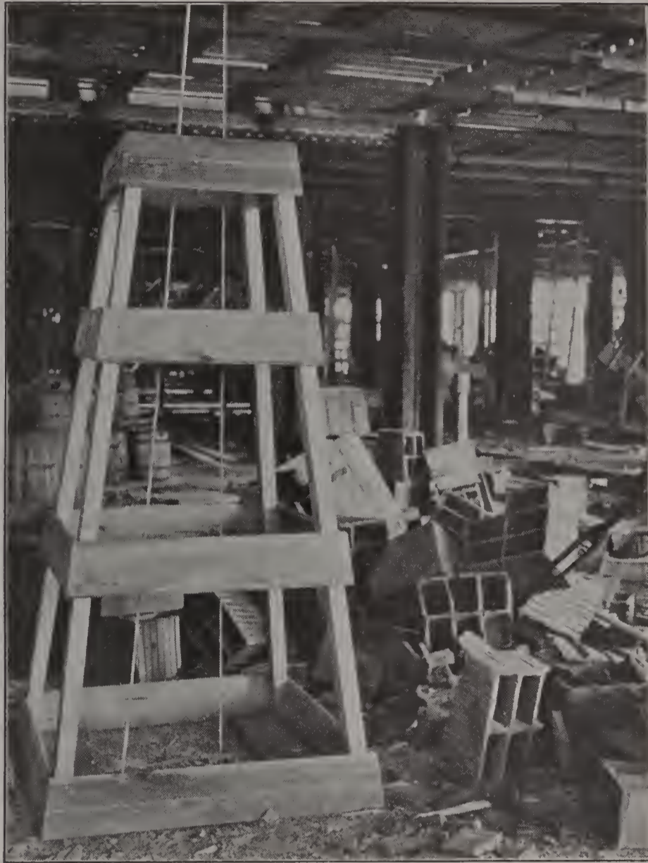
FIG. 11. PROTECTION FOR THE SIGNAL CORDS.
