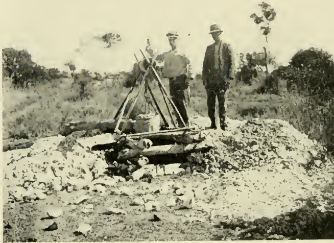
A Lightning Ridge Opal Mine, showing the mouth of the shaft and the windlass by which the broken rock is hauled to the surface.
