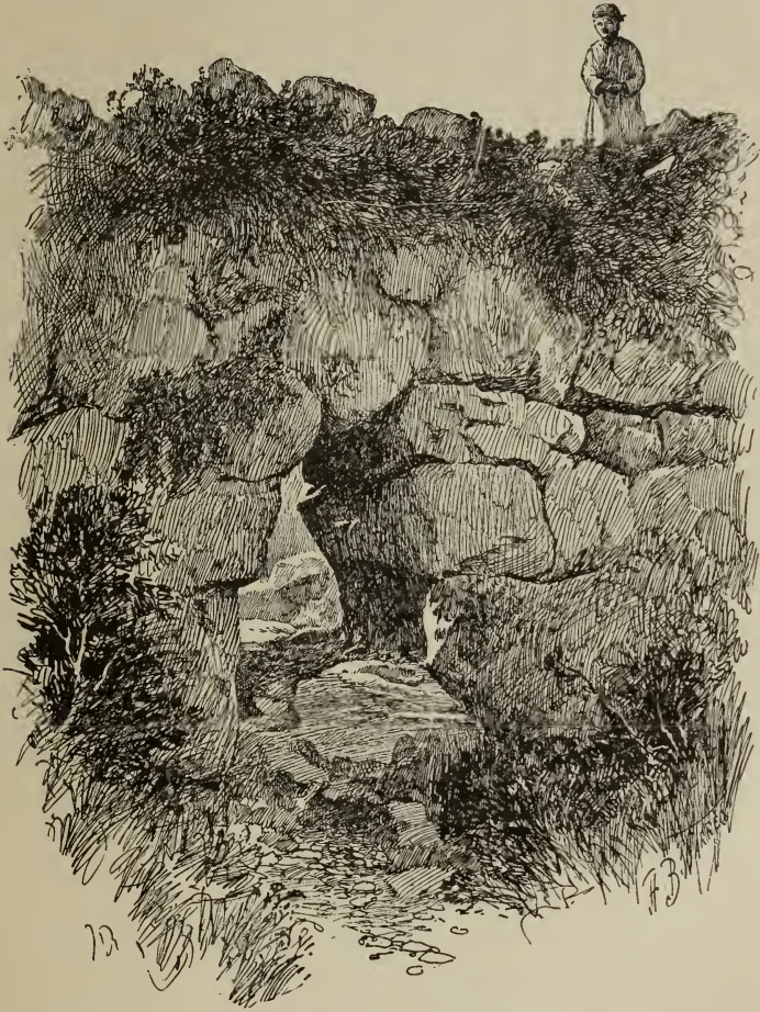
Fig. 9. Cyclopean Bridge near Epidaurus
