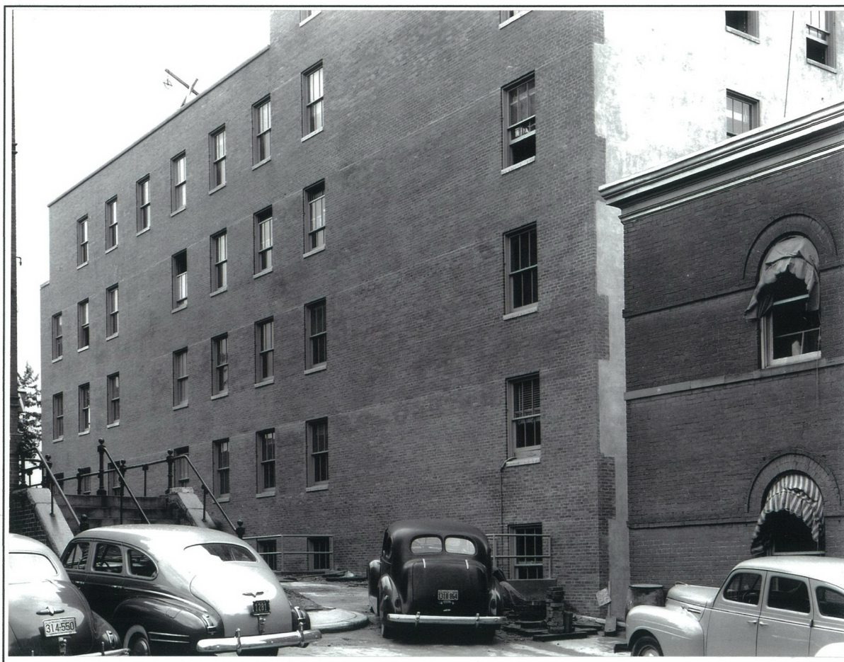
Figure 3. The rear of the new building. Picture taken from the small parking lot to the east of the Ferguson Building. Note the construction of the end of the Old Annex matches that in other pictures. The east end of the new building is not bricked in the same way as the rest of the building, indicating that it was expected to build on to that end (see main text and photo). The five stories are shown, the parking lot being a bit higher than M Street in front, so the rear windows are partially below ground level. A partial 6 th floor also existed (also see Fig. 1).
