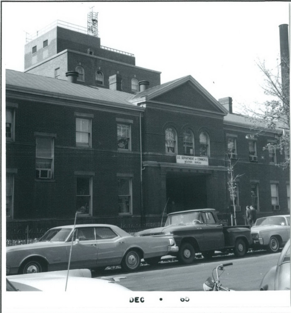
Figure 4. The entrance to the parking lot through the Old Annex from 24 th Street NW. Note the sign “US DEPARTMENT OF COMMERCE WEATHER BUREAU.” The taller building in the background is the new building.
