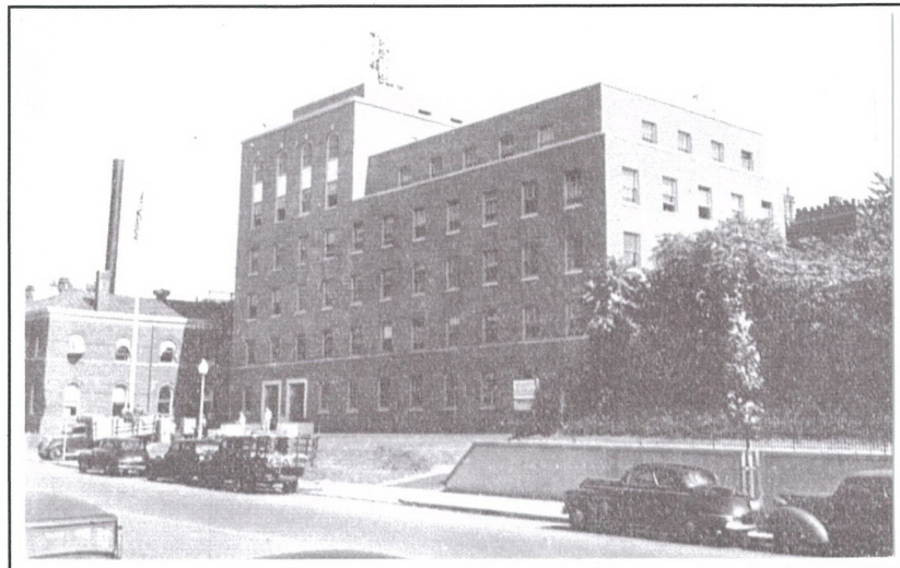
Figure 8. The new building nearing construction with the Old Annex to the left. (Picture taken from July 1941 Weather Bureau Topics and Personnel .)
