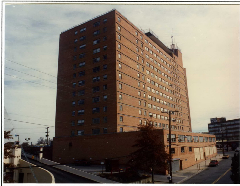
Figure 14. The Kennett Street side (right side of picture) and back of the Gramax Building. Taken from the top of the Montgomery County parking garage, looking southeast. (Photo by Bob Glahn, 1989)
