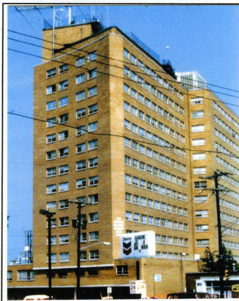
Figure 15. The front and south sides of the Gramax Building. (Picture from the NOAA Library.)
