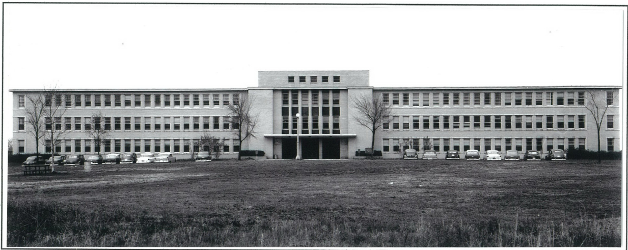
Figure 12. Federal Office Building No. 4 in Suitland, Maryland. Picture taken facing east.
