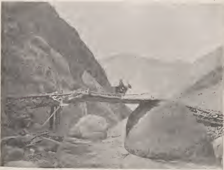
BRIDGE OVER THE GHEZ-DARIA
