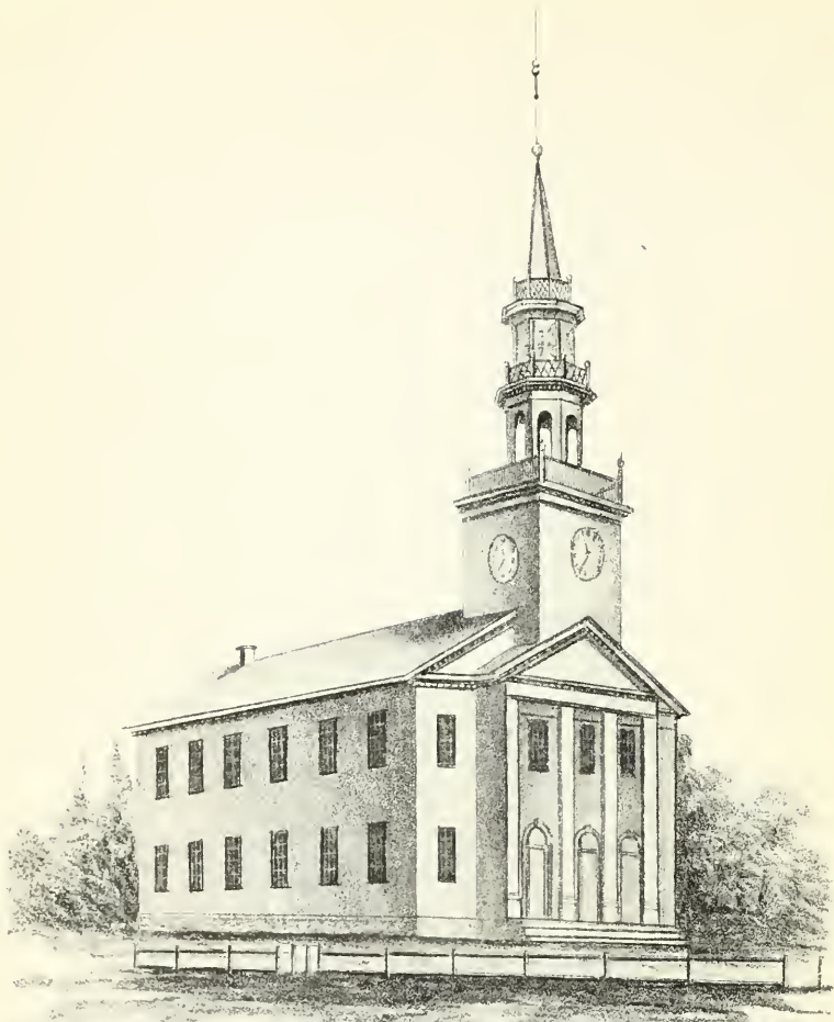
SECOND EDIFICE OF THE FIRST CHURCH OF CHRIST. BUILT IN 1822.
