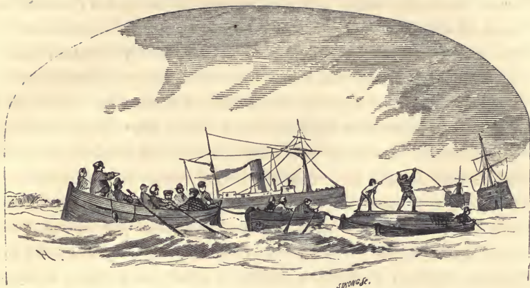
TAKING THE CABLE ASHORE.
