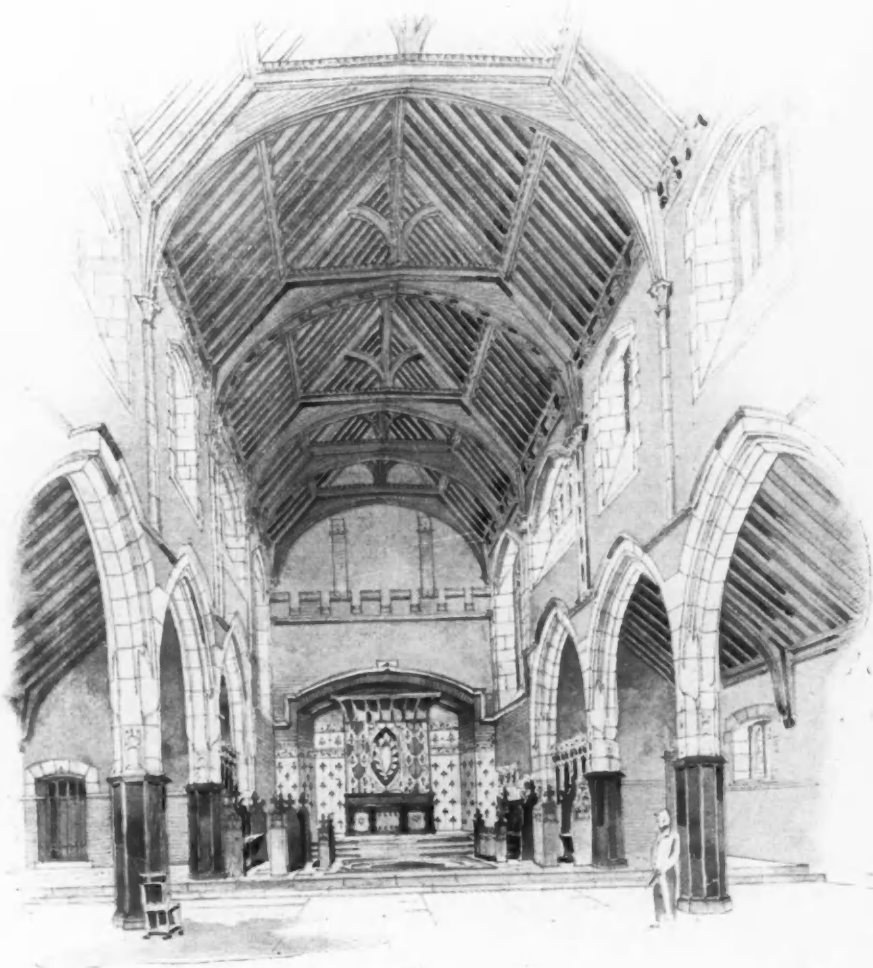
1781. New Church of St. Stephen, Nottingham , WILLIAM D. CARÖE, M.A., Architect.
