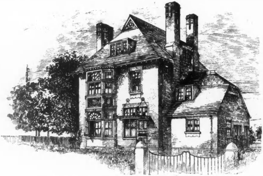
"Claypatch," The Ridgeway, Enfield , SYDNEY W. CRANFIELD, A.R.I.B.A., Architect. (For Plans, see p. 81.)
