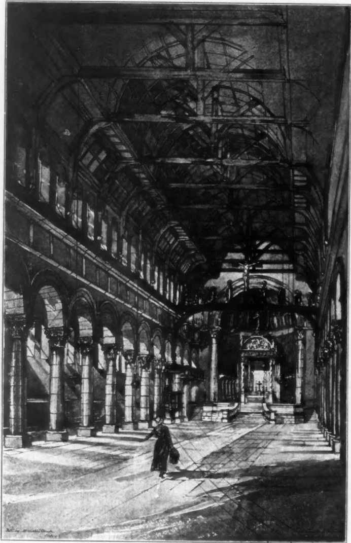
1903. Interior, St. Aidan's Church, Leeds, A. CRAWFORD HICK, Architect.
