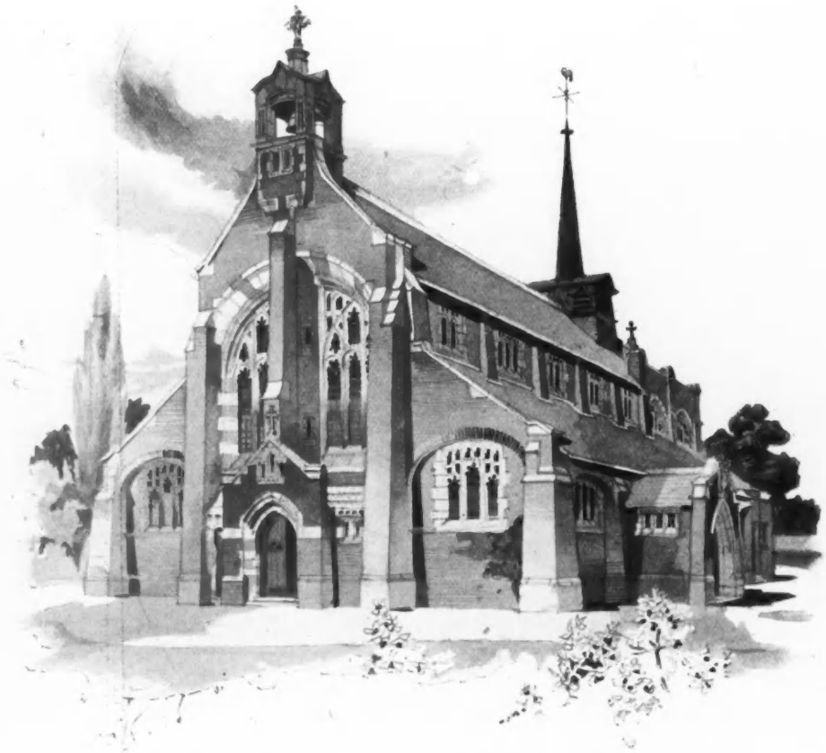
1781. New Church of St. Stephen, Nottingham, WILLIAM D. CARÖE, M.A., Architect.
