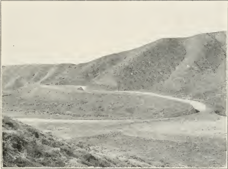
PLATE II.—Main south canal, Uncompahgre Valley. Lined canal section through clay foothills.
