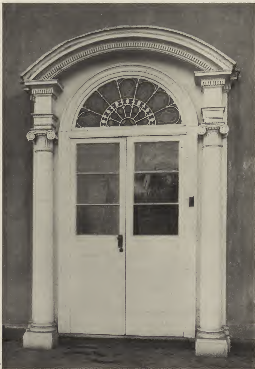
NORTH DOOR—THE WOODLANDS, PHILADELPHIA. BUILT ABOUT 1770. AN EXAMPLE OF THE "THIRD TYPE" OF GEORGIAN.
