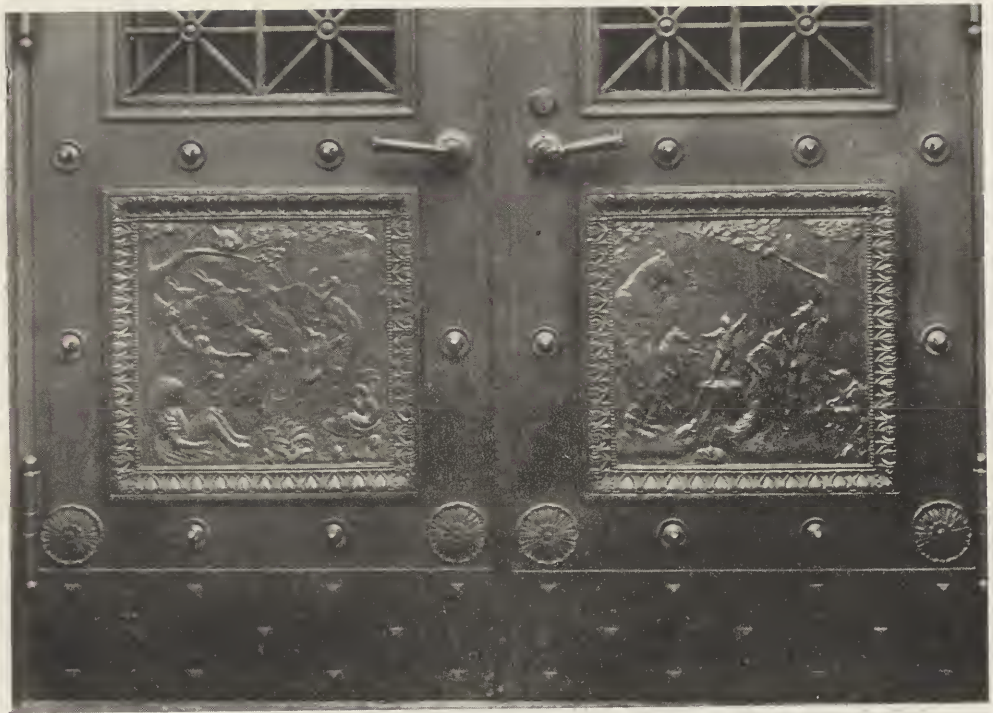
PANELS ON DOORS OF CHILDREN'S ENTRANCE—FORSYTH DENTAL INFIRMARY FOR CHILDREN, BOSTON.
