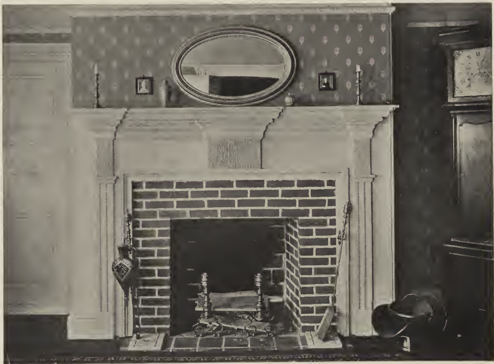
MANTEL DETAIL—TYPICAL OLD SMALL HOUSE, PHILADELPHIA.
