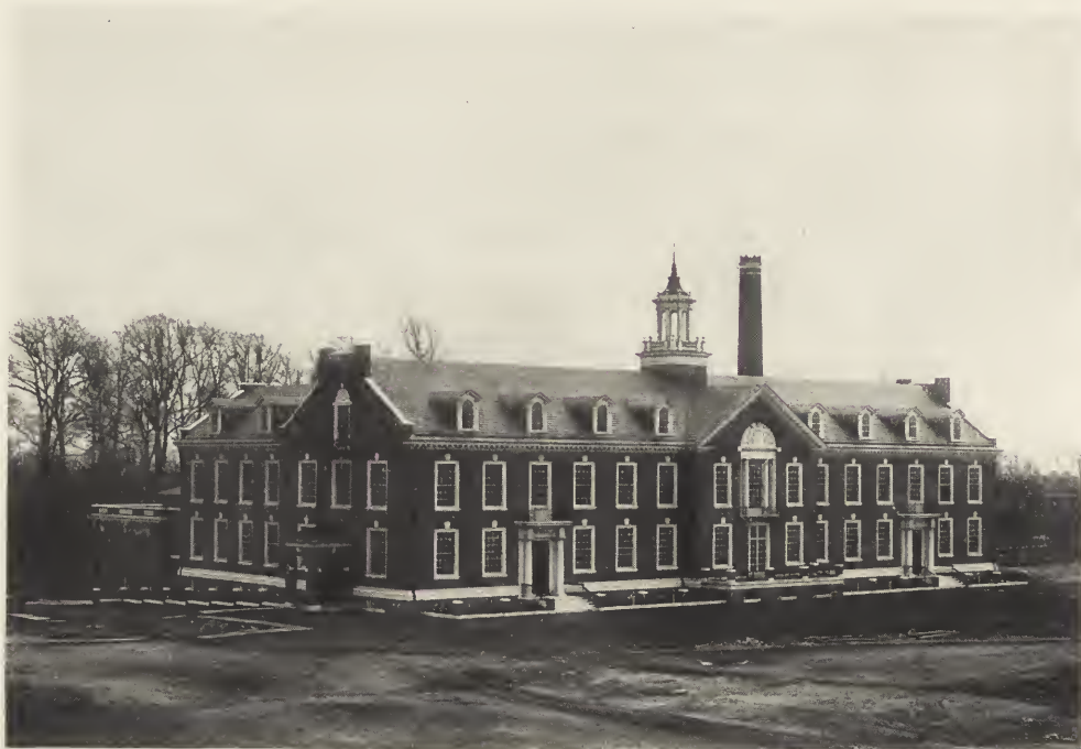
MECHANICAL AND ELECTRICAL ENGINEERING BUILDING, JOHNS HOPKINS UNIVERSITY, HOMEWOOD, BALTIMORE.
