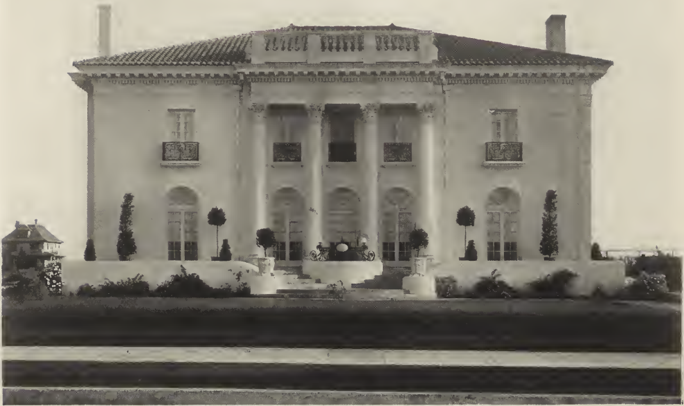
RESIDENCE OF MRS. LOUISE A. DENKER, LOS ANGELES, CAL. B. Cooper Corbett, Architect.
