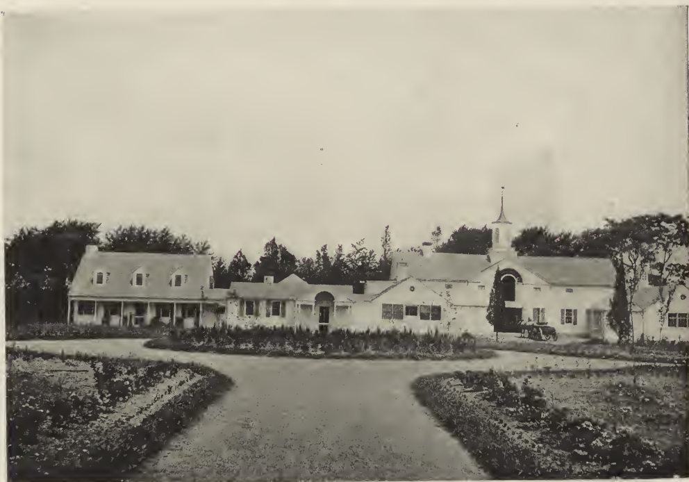
FARM BUILDINGS AND FARMER'S COTTAGE—ESTATE OF C. V. BROKAW, ESQ., GLEN COVE, L. I. Alfred Hopkins, Architect.
