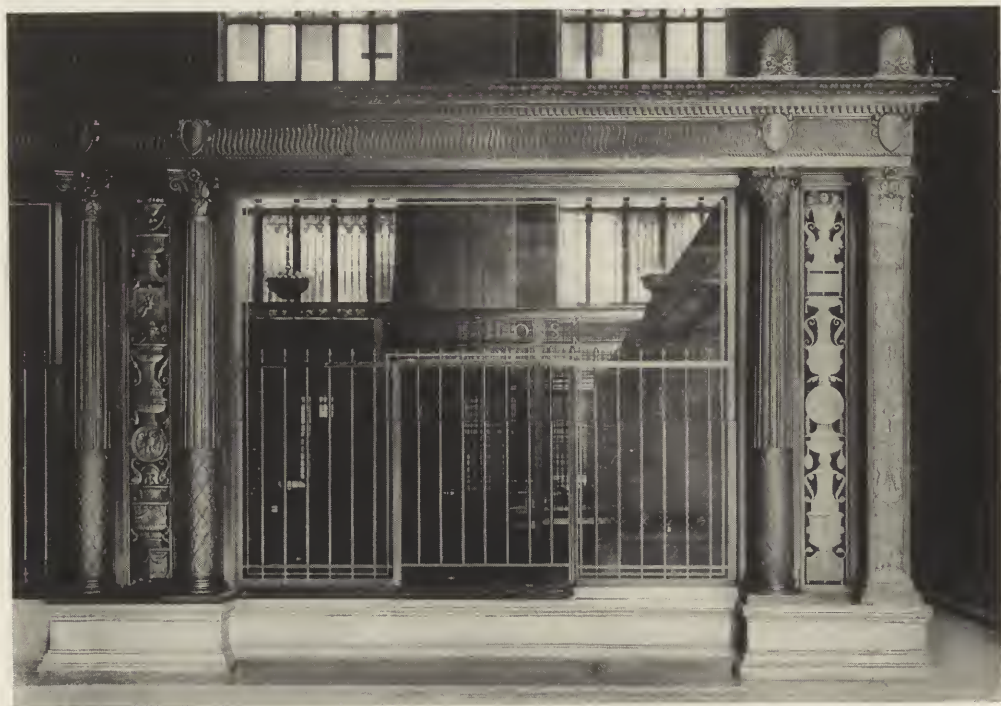
DETAIL OF BRONZE SCREEN—BANKING ROOM, GUARANTY TRUST CO., NEW YORK CITY. York & Sawyer, Architects.
