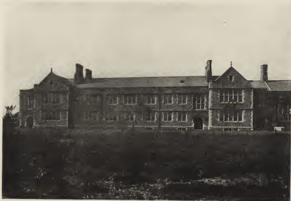
EADS HALL—WASHINGTON UNIVERSITY, ST. LOUIS, MO. Cope & Stewardson, Architects.
