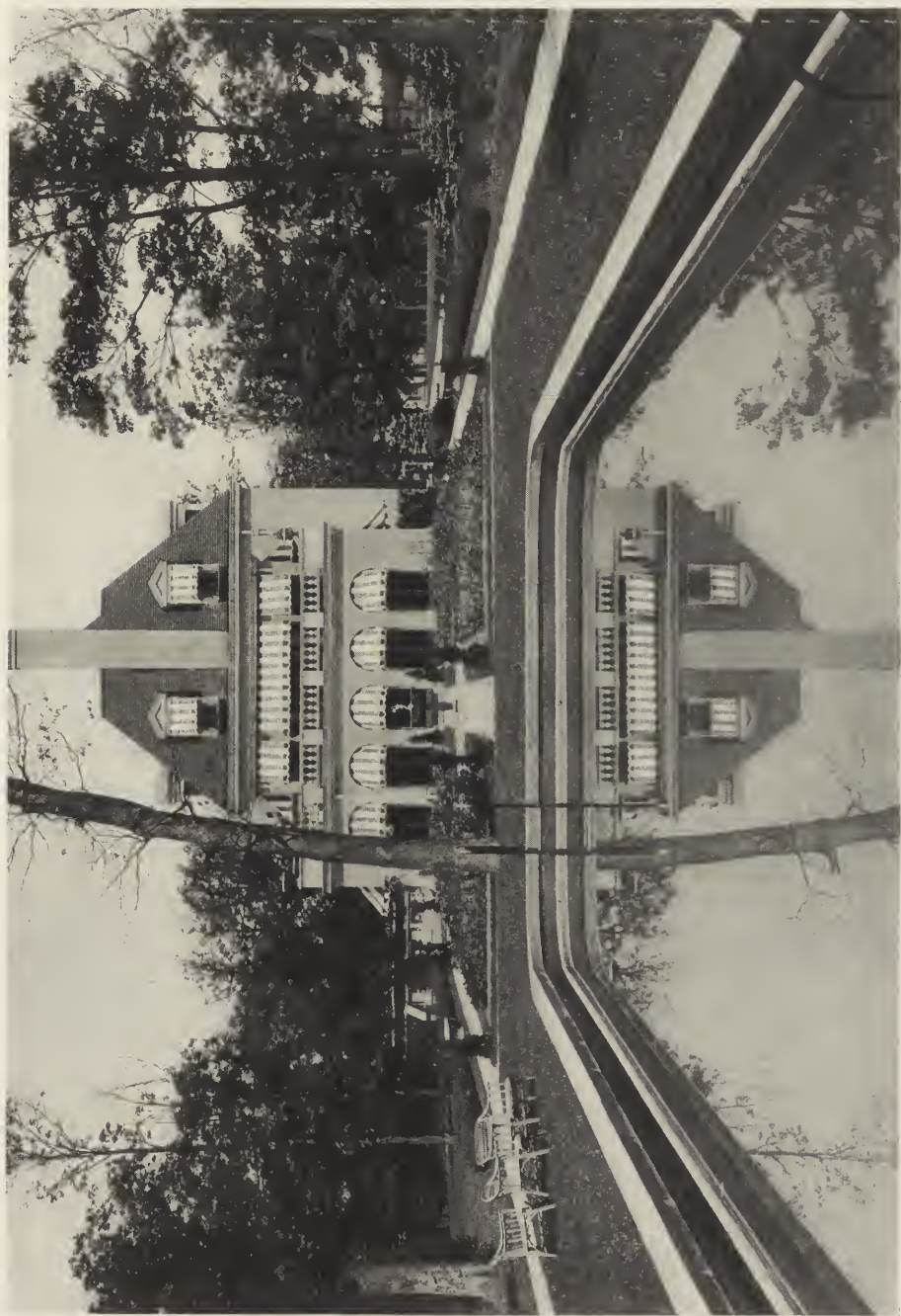
RESIDENCE OF JAMES W. THORNE, ESQ., LAKE FOREST, ILL. OTIS & CLARK, ARCHITECTS.
