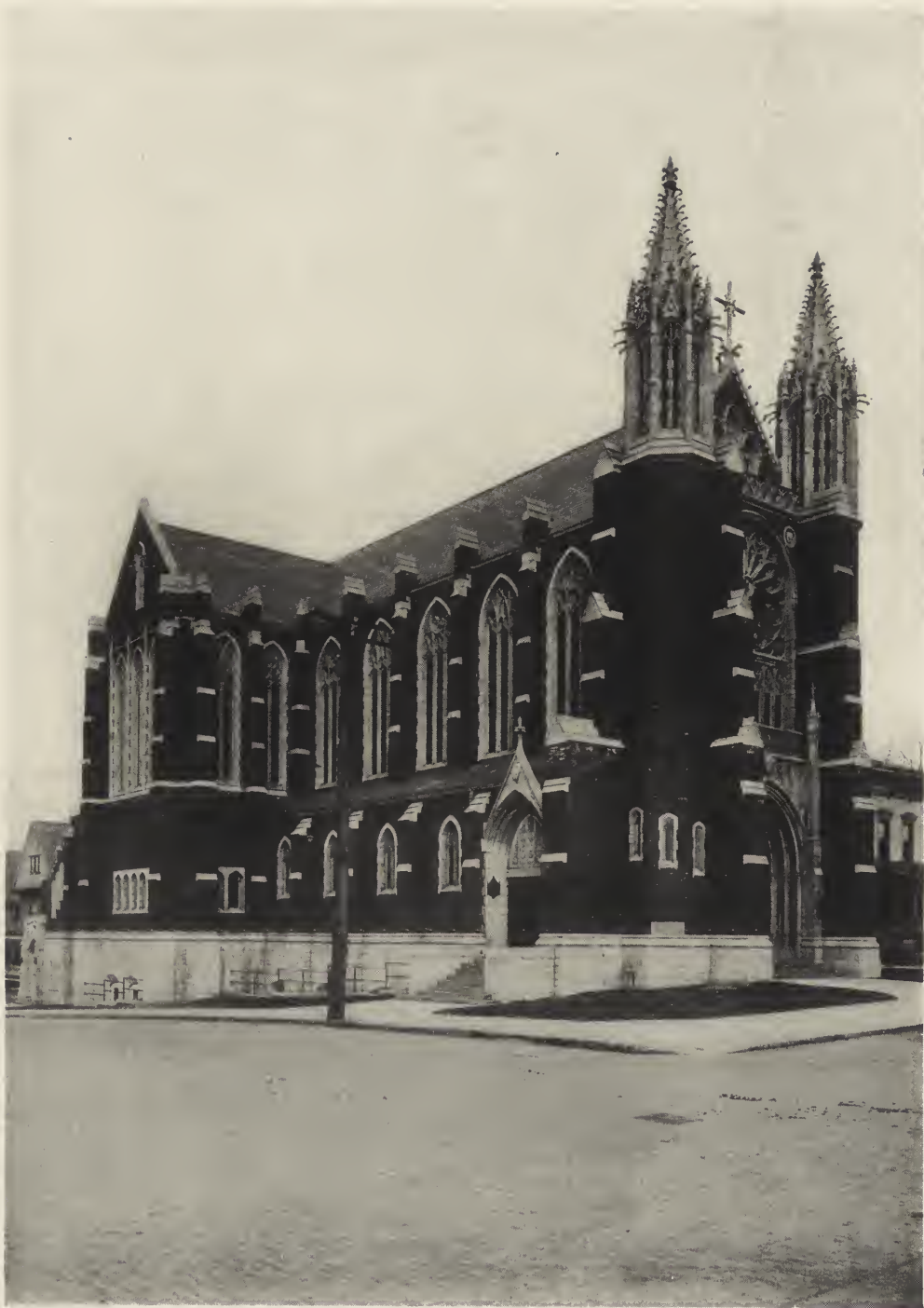
SIDE VIEW—TRINITY LUTHERAN CHURCH, AKRON, OHIO. J. W. C. CORBUSIER, ARCHITECT.
