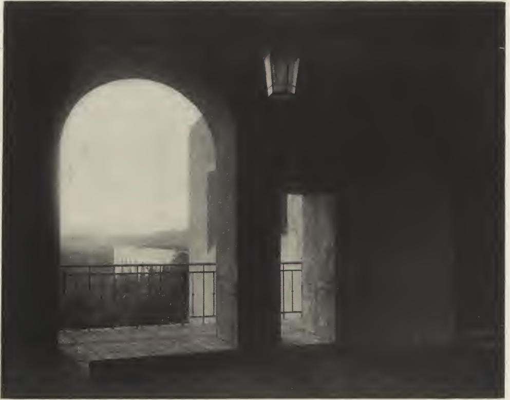
LOOKING OUT ALONG THE CABRILLO BRIDGE FROM A LOGGIA OF THE FINE ARTS BUILDING (PERMANENT)—SAN DIEGO EXPOSITION.
