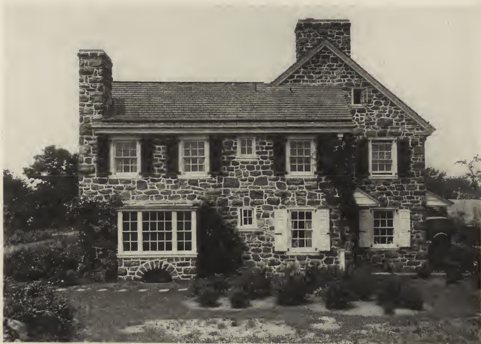
SIDE VIEW—HOUSE OF WILLIAM T. HARRIS, ESQ., VILLA NOVA, PA. Duhring, Okie & Ziegler, Architects.
