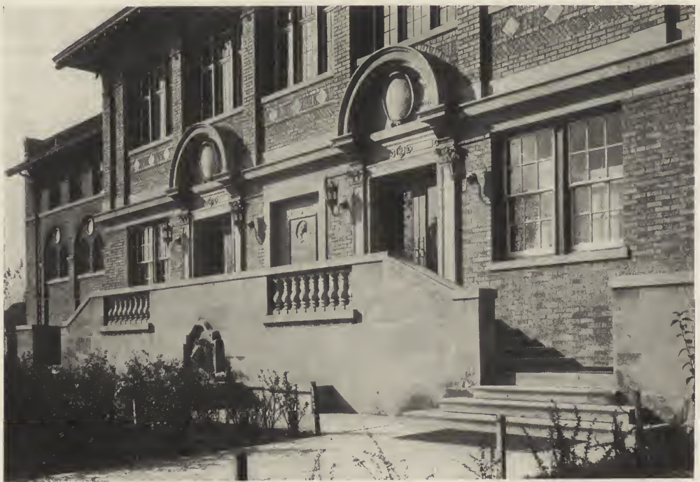
ALLEN STREET ENTRANCE—JOHN C. PROCTOR RECREATION CENTER, PEORIA, ILL. Hewitt & Emerson, Architects.
