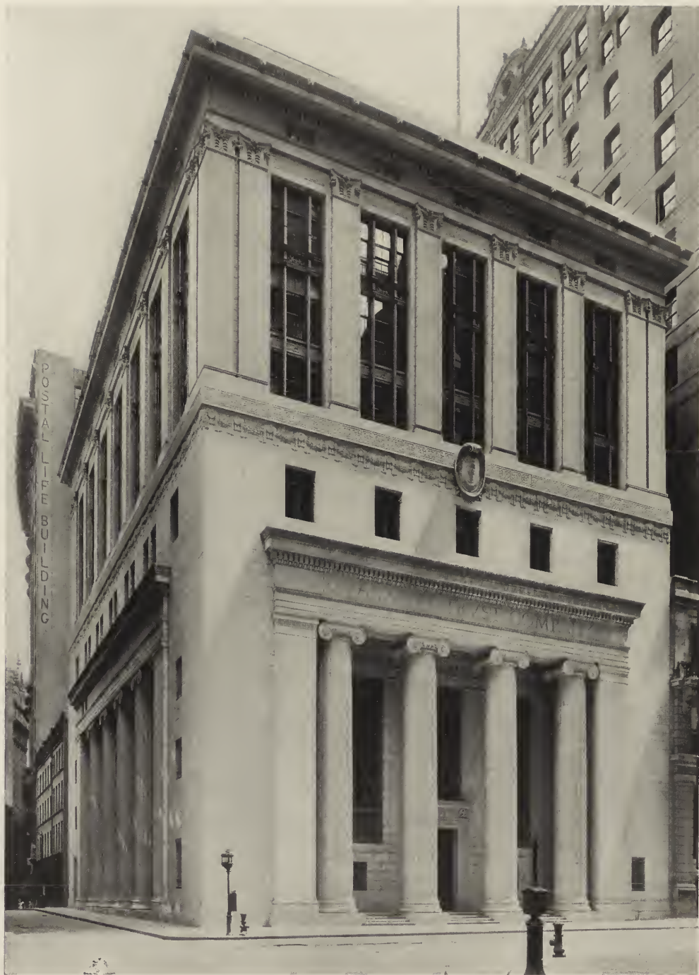
BANKING HOUSE OF THE GUARANTY TRUST COMPANY, NEW YORK CITY. YORK & SAWYER, ARCHITECTS.
