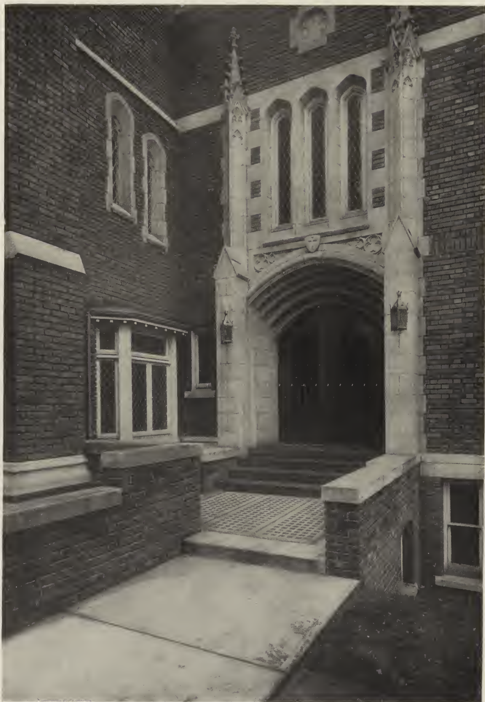
SUNDAY SCHOOL ENTRANCE—TRINITY LUTHERAN CHURCH, AKRON, OHIO. J. W. C. CORBUSIER, ARCHITECT.
