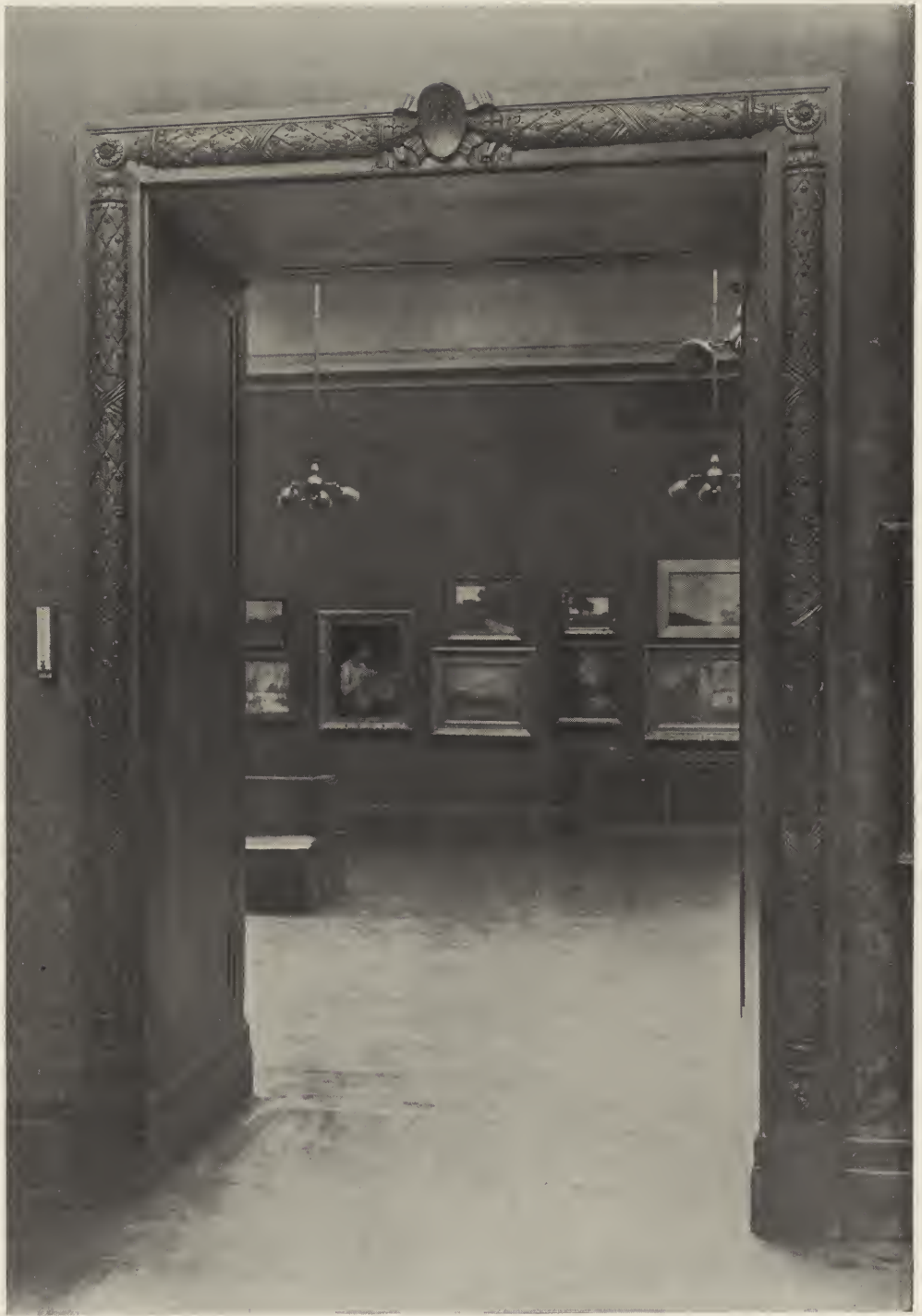
DOORWAY TO EXHIBITION GALLERIES—MONTREAL ART GALLERY. E. AND W. S. MAXWELL, ARCHITECTS.
