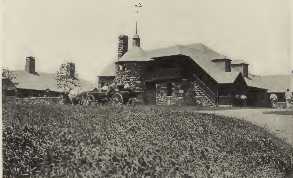
MEN'S QUARTERS, FARM BUILDINGS—ESTATE OF HENRY M. TILFORD, ESQ., MONROE, N. Y. Alfred Hopkins, Architect.
