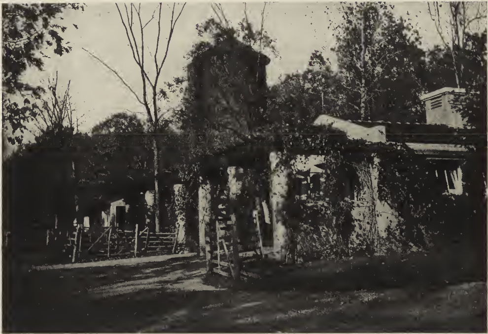
COW BARN AND SILO—ESTATE OF FRANCIS LYNDE STETSON, ESQ., STERLINGTON, N. Y. Alfred Hopkins, Architect.
