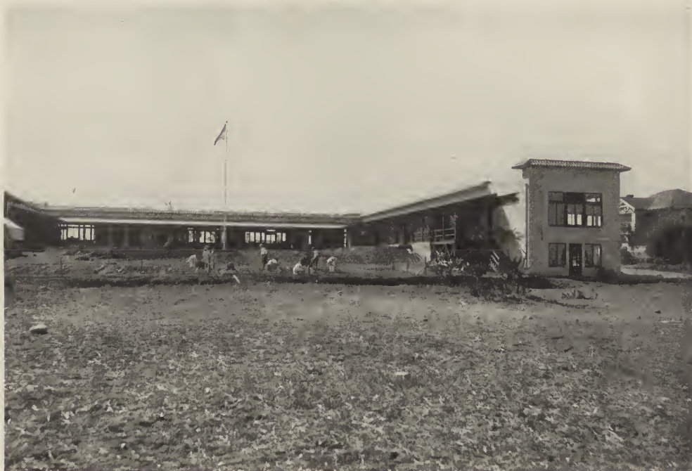
SOUTH AND WEST WINGS—FRANCIS W. PARKER SCHOOL OF SAN DIEGO. Wm. Templeton Johnson, Architect.
