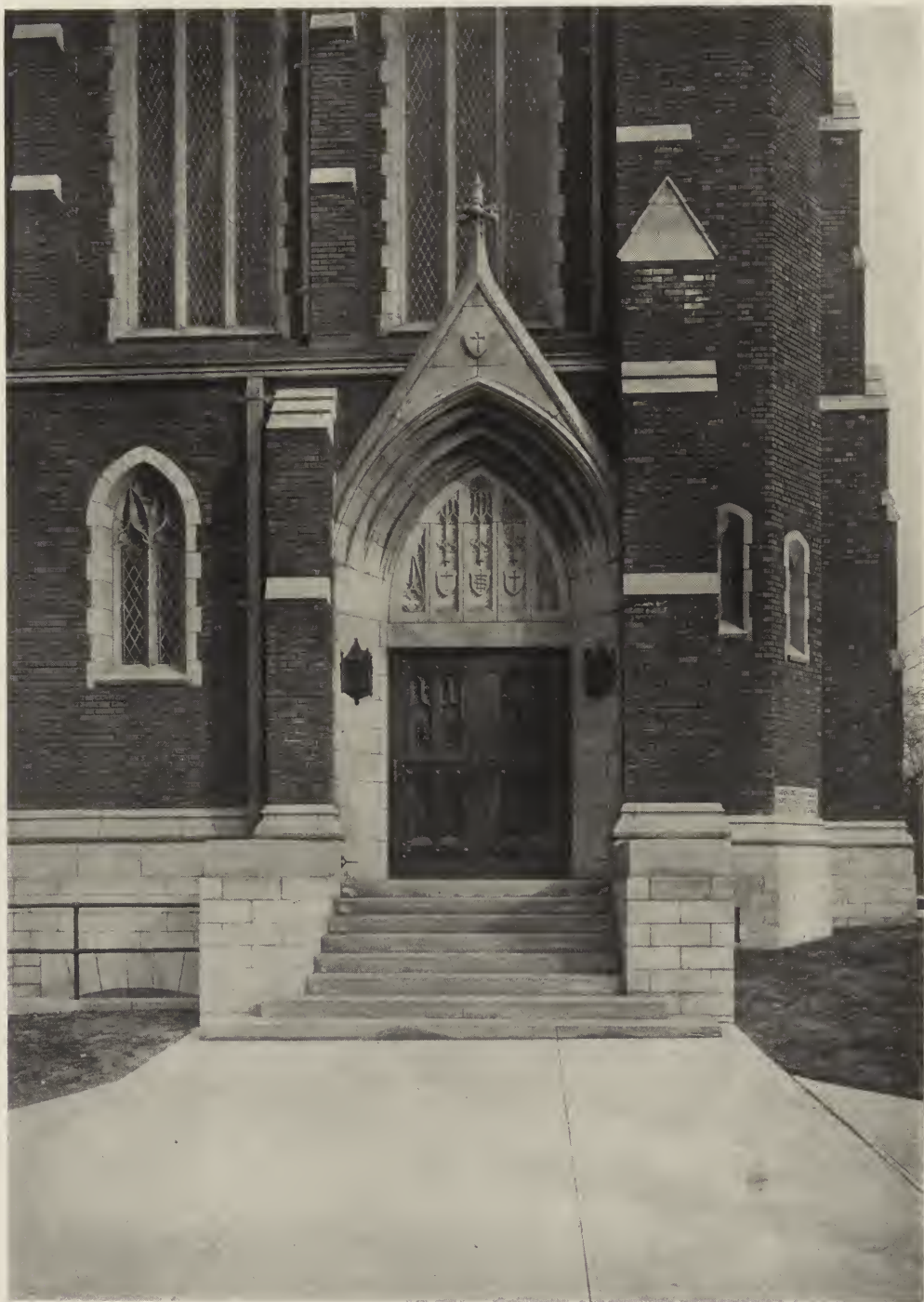
NARTHEX SIDE ENTRANCE—TRINITY LUTHERAN CHURCH, AKRON, OHIO. J. W. C. CORBUSIER, ARCHITECT.
