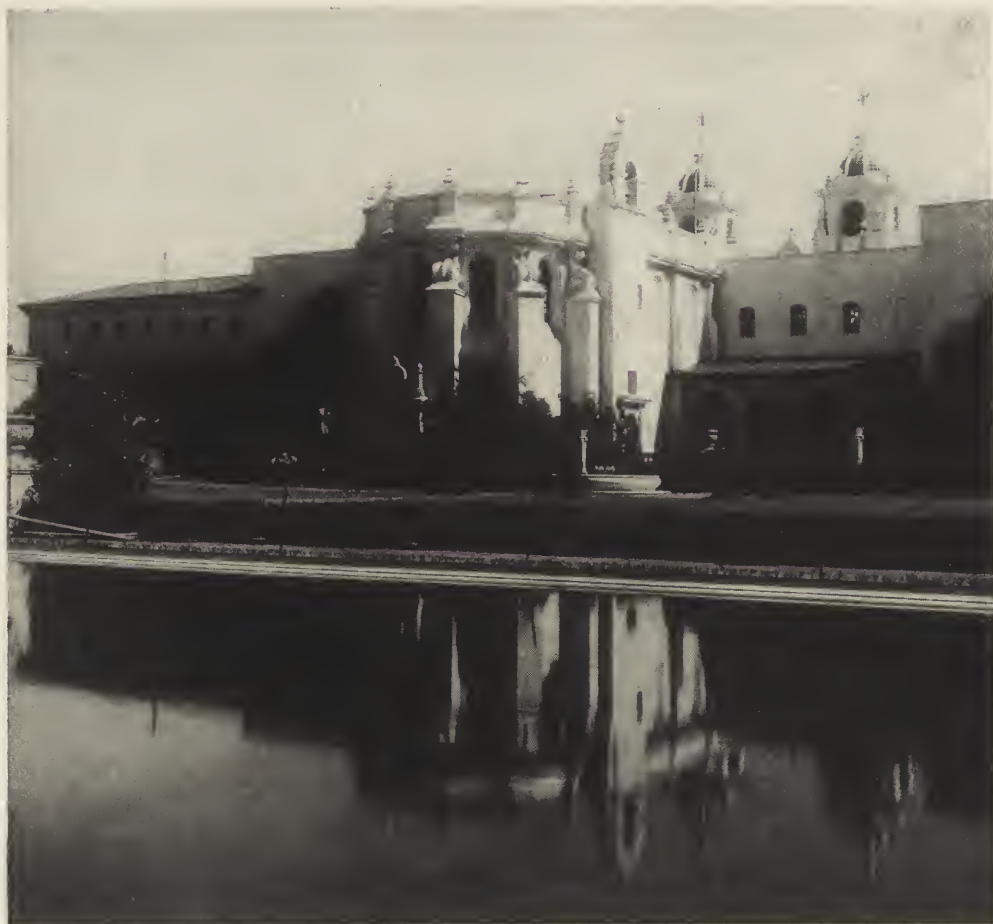
COMMERCE AND INDUSTRIES BUILDING, ACROSS THE LAGOON OF FLOWERS, SAN DIEGO EXPOSITION.
