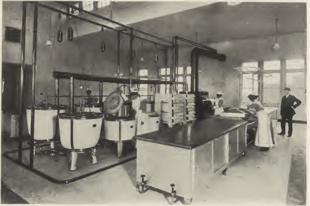
KITCHEN—THE NEW GENERAL HOSPITAL, CINCINNATI, OHIO. Samuel Hannaford & Sons, Architects.
