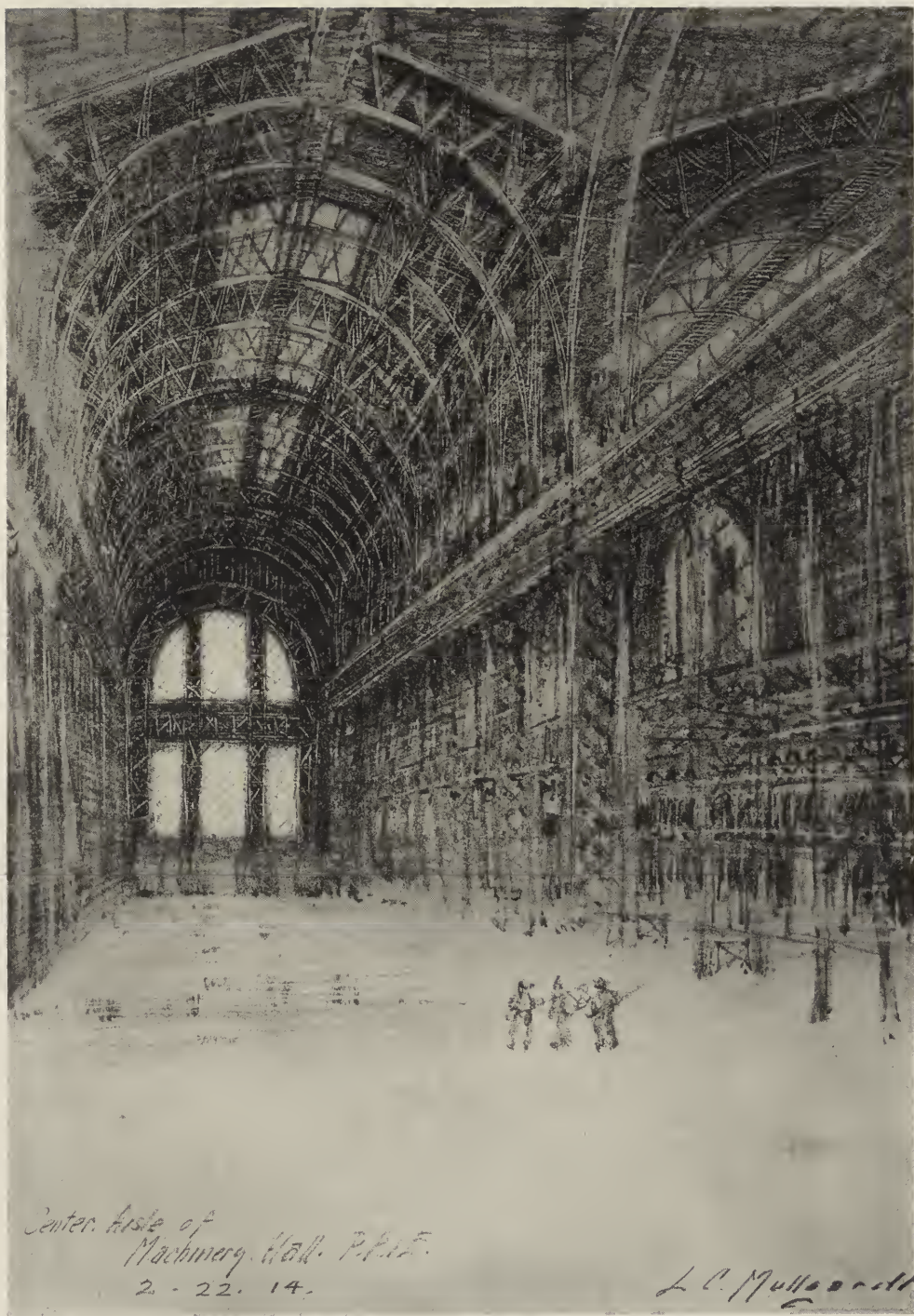
SKETCH SHOWING INTERIOR CONSTRUCTION OF PALACE OF MACHINERY, FEBRUARY, 1914. DESIGNED BY THE ENGINEERING DEPARTMENT OF THE PANAMA-PACIFIC EXPOSITION. WARD & BLOHM, ARCHITECTS.
