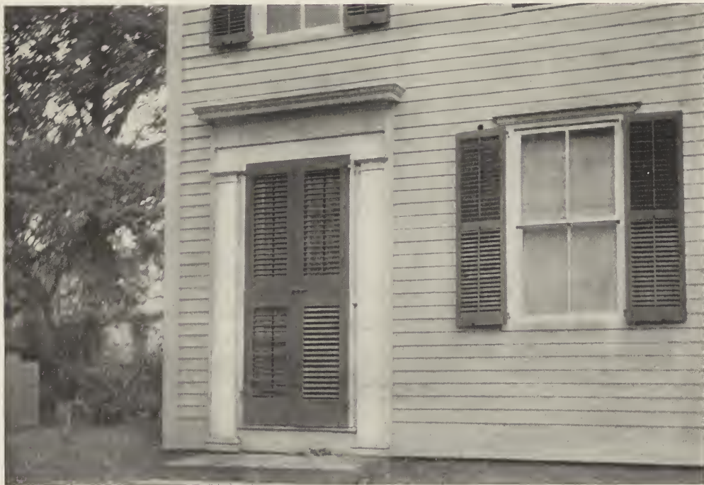
TYPICAL DOORWAY OF SMALL HOUSE OF THE PERIOD OF THE CLASSIC REVIVAL.
