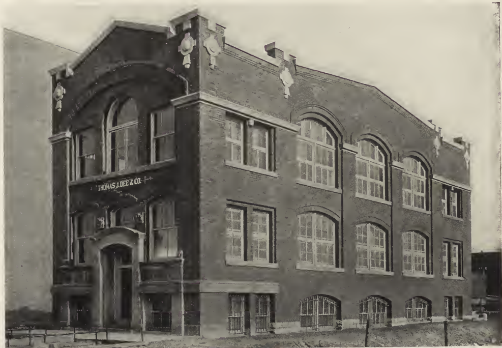
LABORATORY OF THOS. J. DEE & CO., CHICAGO. Hill & Woltersdorf, Architects.
