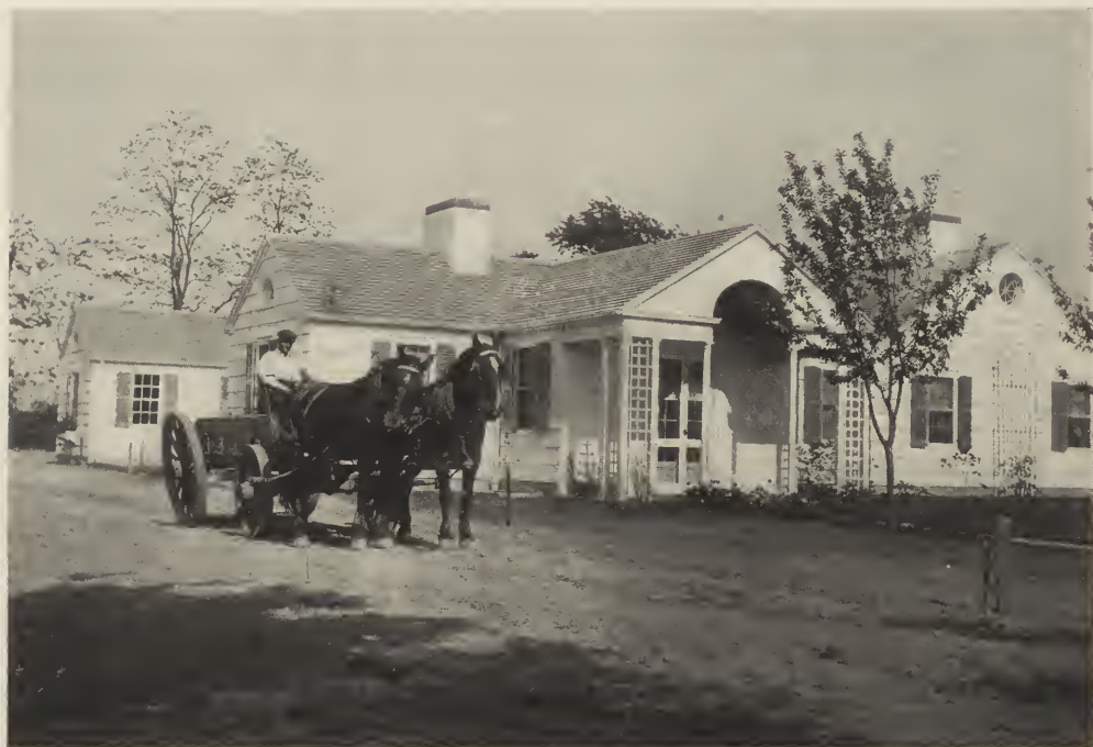
FARM BUILDINGS—ESTATE OF MRS. GLENN STEWART, LOCUST VALLEY, L. I. Alfred Hopkins, Architect.
