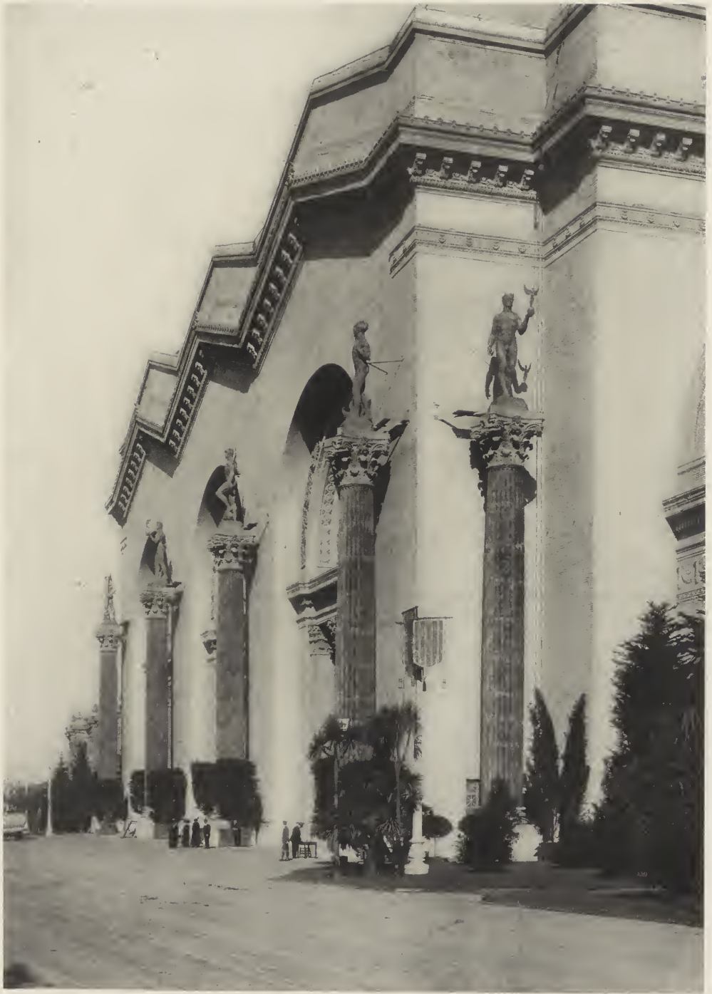
CENTRAL PORTION OF THE WEST FACADE OF THE PALACE OF MACHIN- ERY. WARD & BLOHM, ARCHITECTS.
