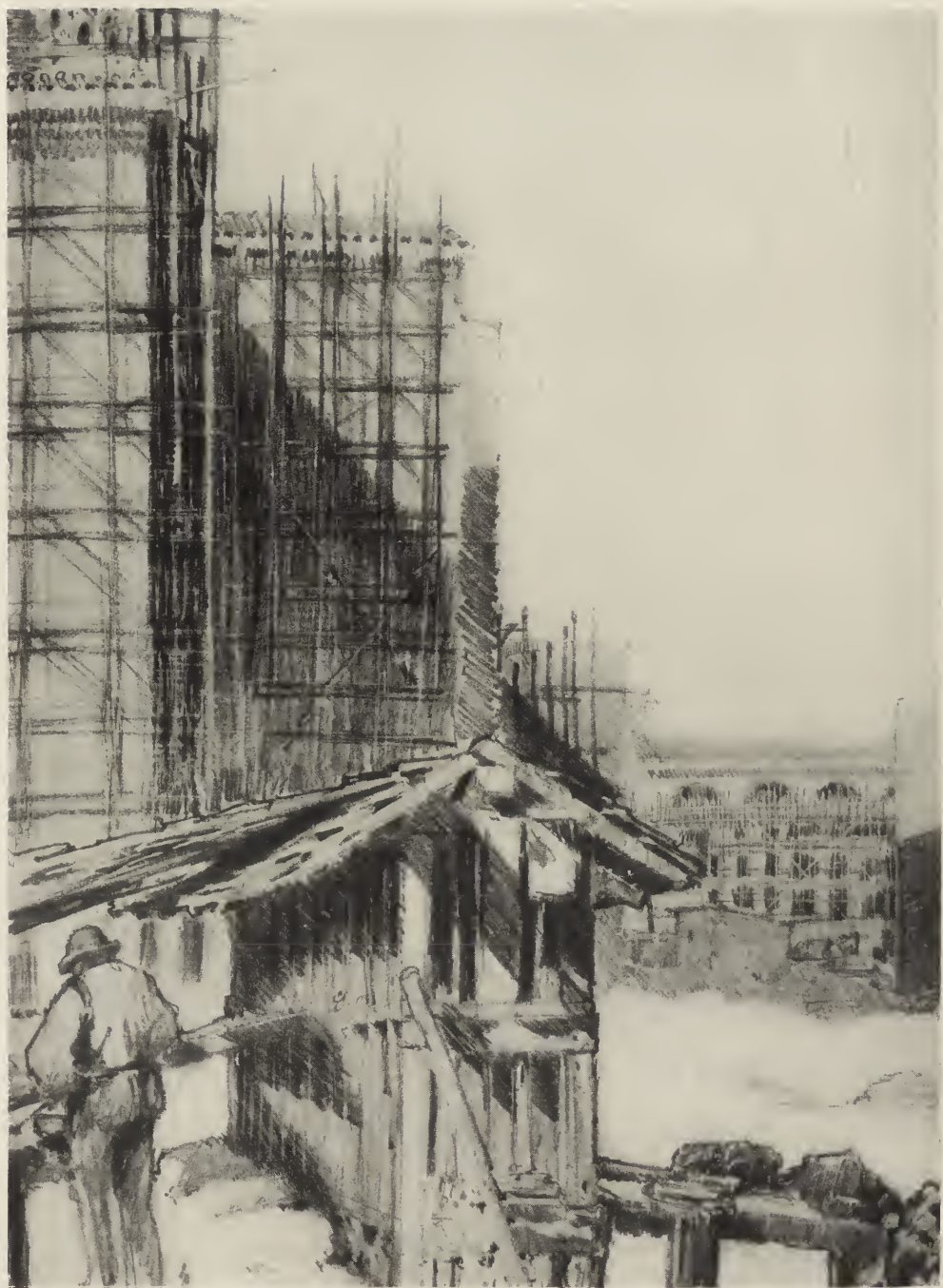
SKETCH OF PRELIMINARY CONSTRUCTION AROUND THE COURT OF PALMS, MARCH, 1914. DESIGNED BY THE ENGINEERING DEPARTMENT OF THE PANAMA-PACIFIC EXPOSITION. GEORGE W. KELHAM, ARCHITECT.
