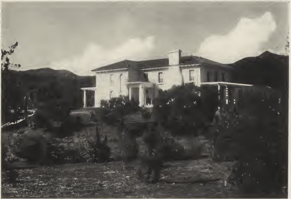
RESIDENCE OF C. F. PERRY, ESQ., HOLLYWOOD, CAL. B. Cooper Corbett, Architect.
