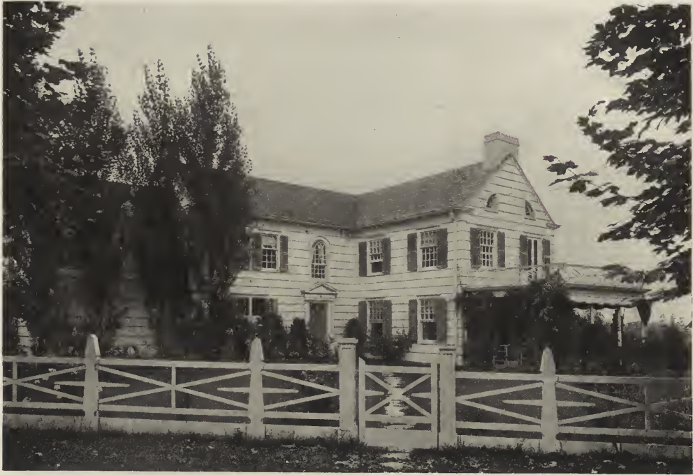
SIDE ENTRANCE—OWN HOUSE, NEW CANAAN, CONN. Electus D. Litchfield, Architect.
