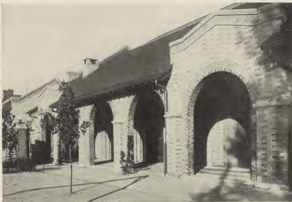
LOGGIA, WOMEN'S GYMNASIUM—JOHN C. PROCTOR RECREATION CENTER, PEORIA, ILL. Hewitt & Emerson, Architects.
