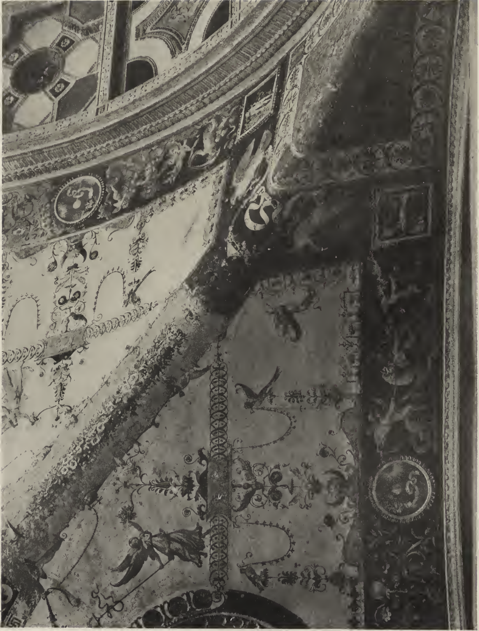
DETAIL OF GROINED VAULT IN LOGGIA—VILLA MADAMA, ROME.
