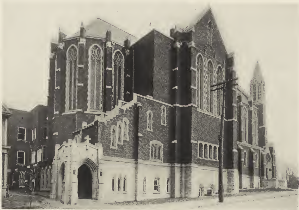
REAR VIEW—TRINITY LUTHERAN CHURCH, AKRON, OHIO. J. W. C. Corbusier, Architect.
