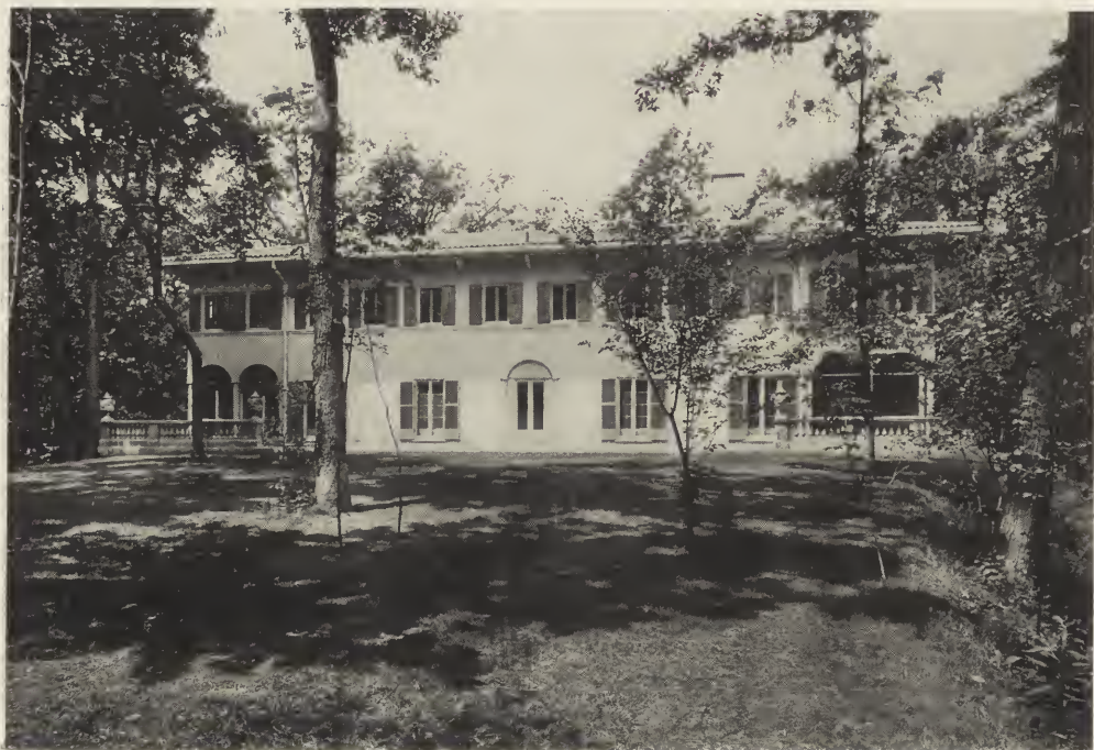
RESIDENCE OF WALTER R. KIRK, ESQ., LAKE FOREST, ILL. Otis & Clark, Architects.
