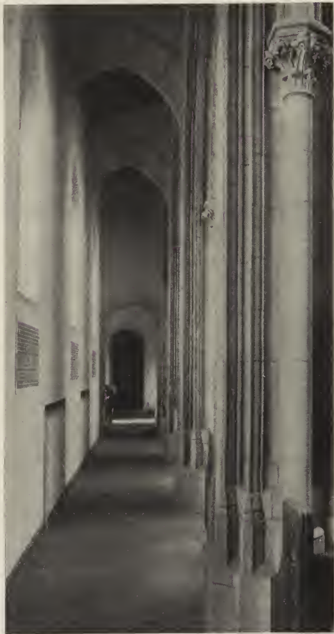
SOUTH SIDE AISLE—TRINITY LUTHERAN CHURCH, AKRON, OHIO.
