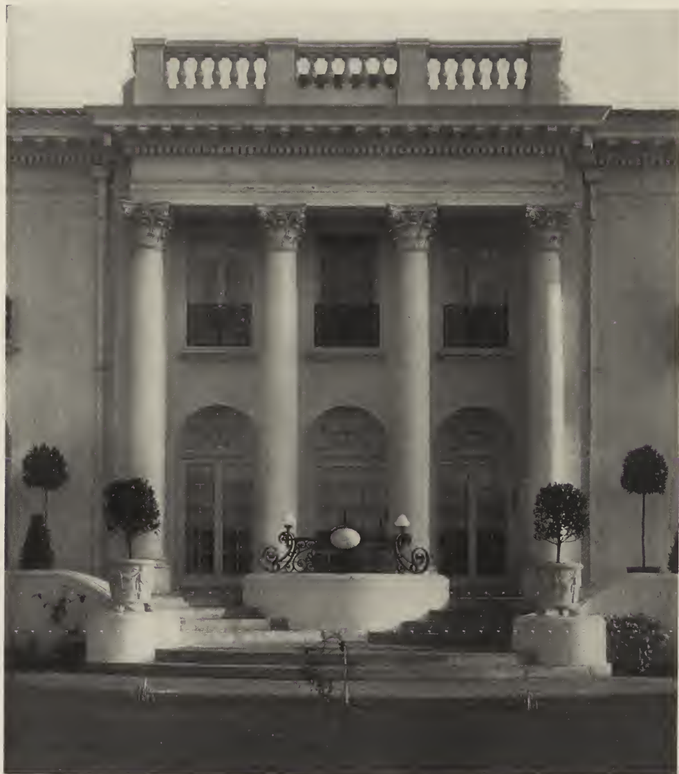
DETAIL—RESIDENCE OF MRS. LOUISE A. DENKER, LOS ANGELES, CAL. B. COOPER CORBETT, ARCHITECT.
