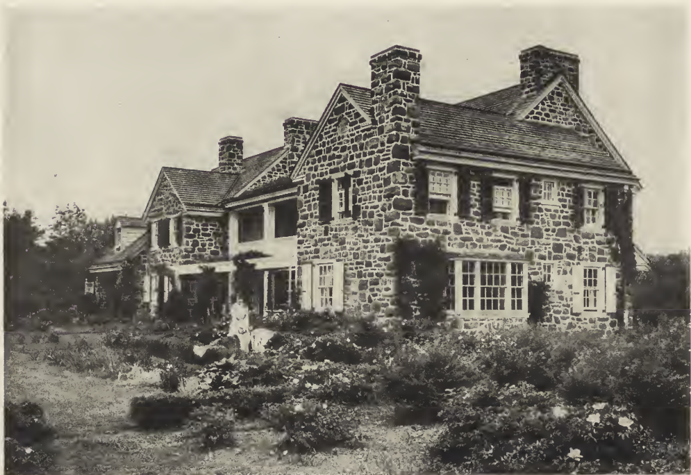
OBLIQUE REAR VIEW—HOUSE OF WILLIAM T. HARRIS, ESQ., VILLA NOVA, PA. Duhring, Okie & Ziegler, Architects.
