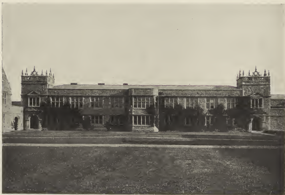
BUSCH HALL—WASHINGTON UNIVERSITY, ST. LOUIS, MO. Cope & Stewardson, Architects.
