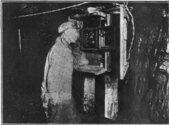
The hoisting engineer takes special orders Mine telephone installation in a coal entry
