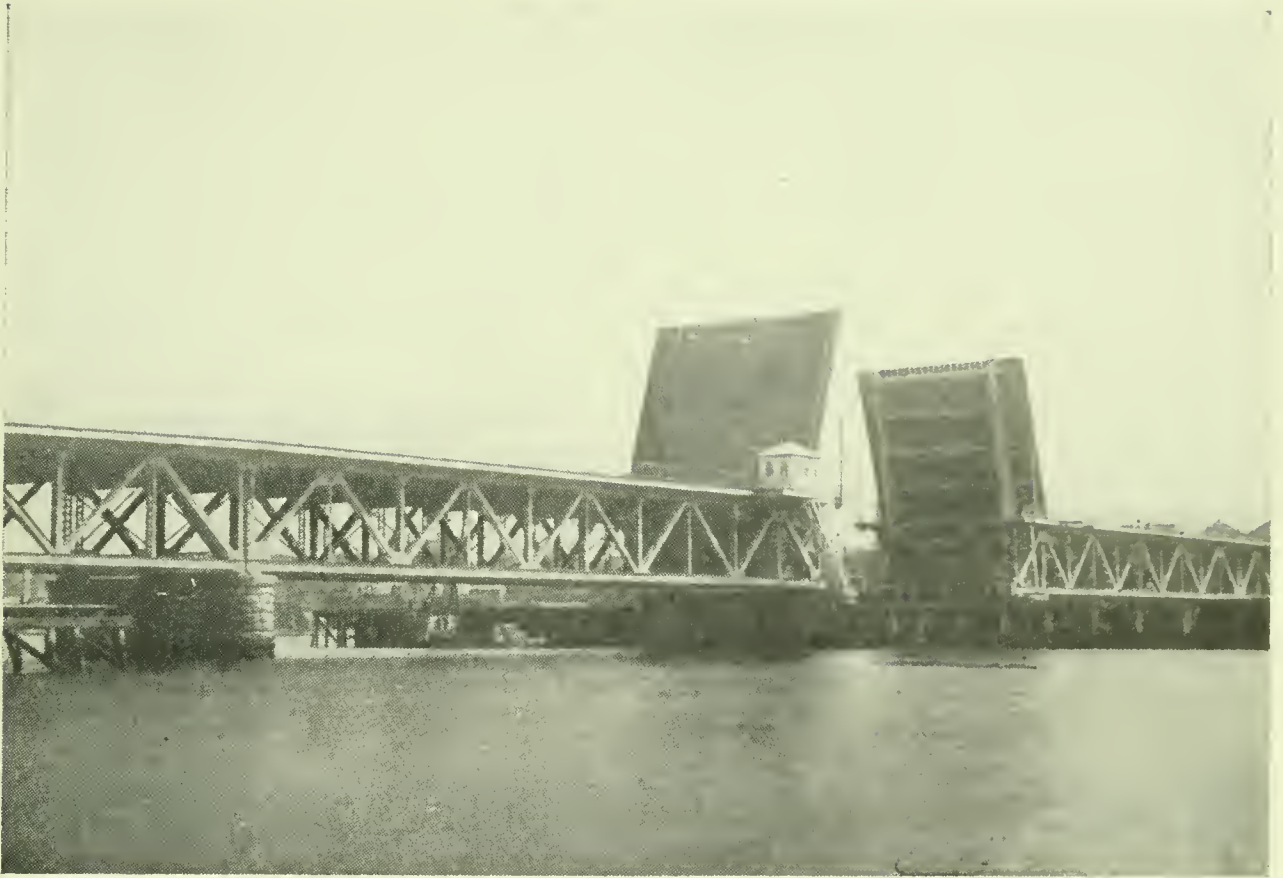
NEW BRIDGE, CROSSING TAUNTON RIVER
