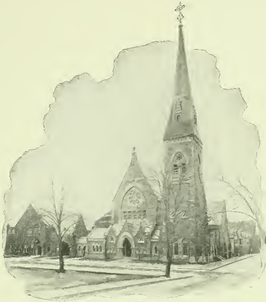
CENTRAL CONGREGATIONAL CHURCH
