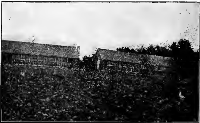
Two well-lighted brooder houses, equipped with individually heated hovers.
