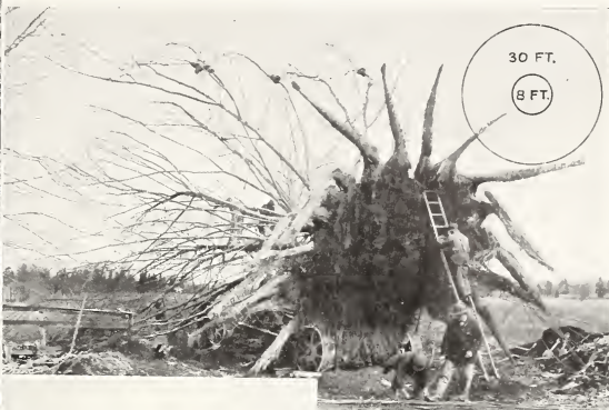
Large English Beech moved for Mr. J.S. Phipps, Westbury, L. I. The large circle shows the Hicks system with large ball of earth in the center and wide spread of small feeding roots outside. The smaller circle shows the frequent method of moving large trees with small area of roots
