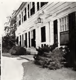
Yew and Juniper at the residence of Mr. George B. Hedges, Westbury; E. G. Davis, Landscape architect, Ithaca, N. Y. let the foundation show in some places.
