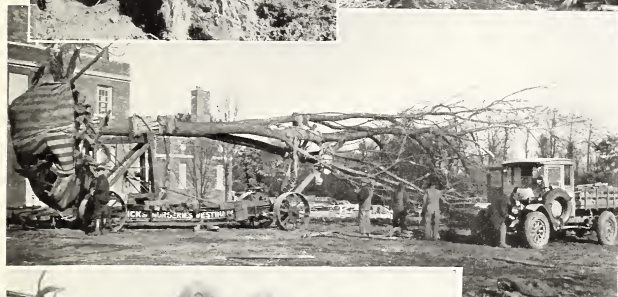
Large English Beech moved for Mr. J.S. Phipps, Westbury, L. I. The large circle shows the Hicks system with large ball of earth in the center and wide spread of small feeding roots outside. The smaller circle shows the frequent method of moving large trees with small area of roots
