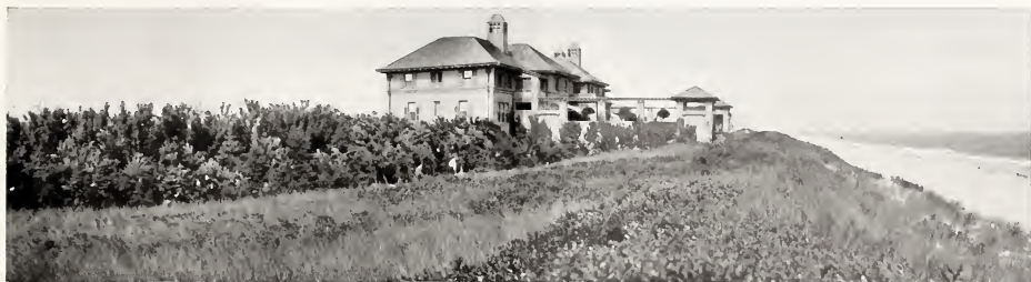
Eight carloads of salt spray resistant Pines from Hicks Nurseries planted here in August to screen an outdoor gymnasium. For trees to stand the severe conditions of the seashore they must learn from the sand dunes. The sand establishes an equilibrium between surf and wind
