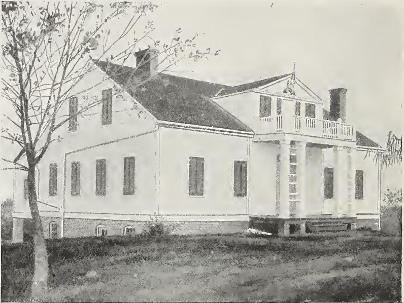
Shirley House after Restoration.
