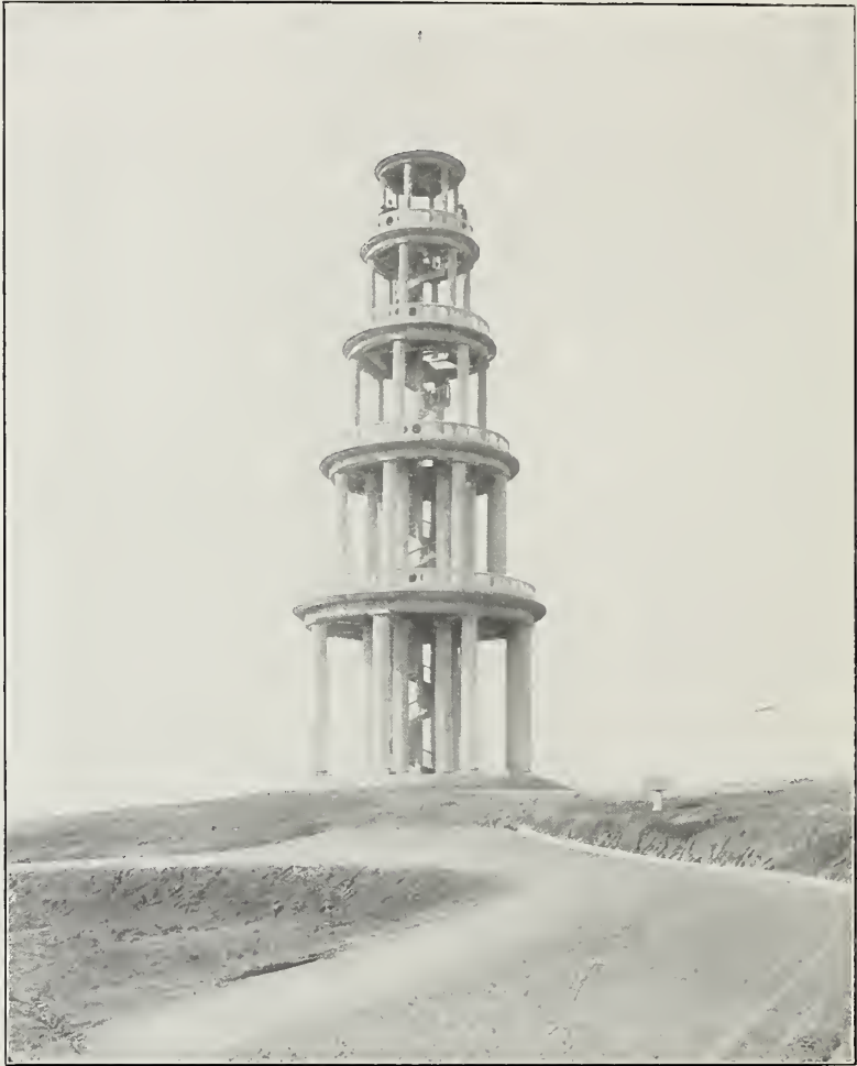
Park Observation Tower, Three of which have been Erected at a cost of $30,000.
