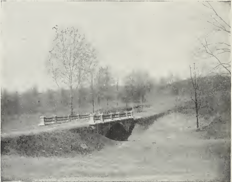
Bridge on Union Avenue.
