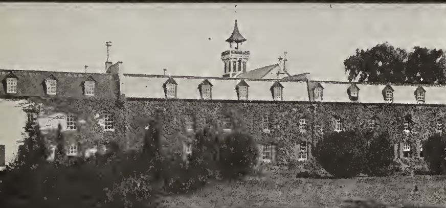
WAREHOUSE AT BLOOMSDALE, 1876
