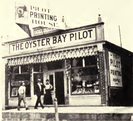
Oyster Bay Pilot Newspaper Office where Mr. Roosevelt's letters of acceptance were ordered printed.
