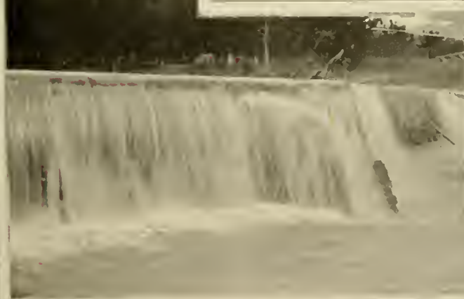
MILL DAM AT CADDO GAP
