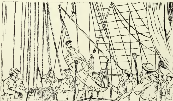
Fig. 6.—("D")—Lowering through the Hatchway.
