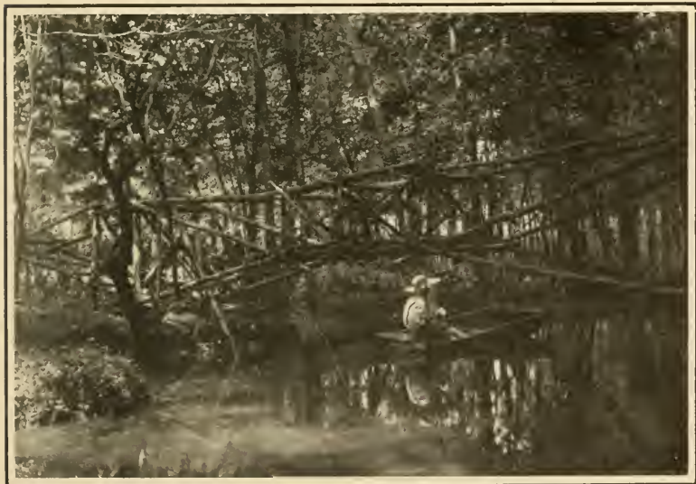
The Cantilever Bridge in Reddy's Back Yard.
