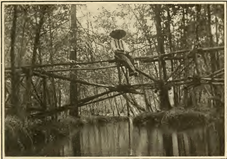
Fishing off the Cantilever Bridge.
