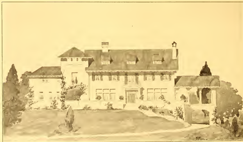
RESIDENCE OF MRS. E. W. IRELAND, AT ROSLYN, L. I. STUEL & BRYSON, ARCHITECTS, BROOKLYN.
