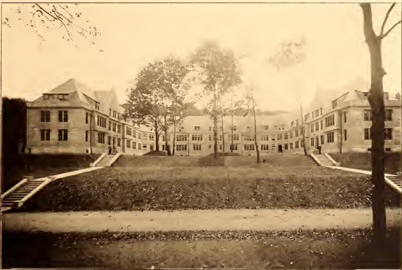
TAYLOR HALL—DORMITORY FOR LEHIGH UNIVERSITY, SOUTH BETHLEHEM, PA. WHITFIELD & KING, Architects, NEW YORK.
