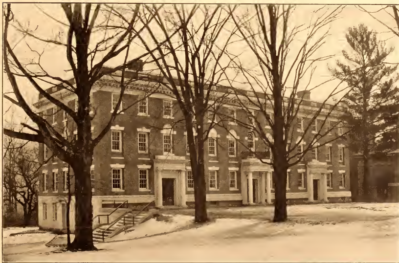
BERKSHIRE DORMITORY, WILLIAMS COLLEGE, WILLIAMSTOWN, MASS. ALLEN & COLLENS, Architects, NEW YORK AND BOSTON.
