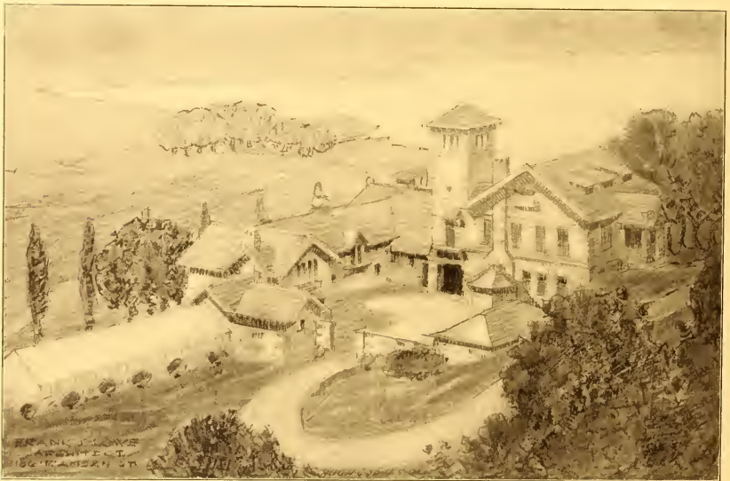
STABLE AND GARDENER'S COTTAGE FOR MESSRS. McLAUGHLIN, RYE, N. Y. FRANK S. LOWE, Architect, BROOKLYN, N. Y.
