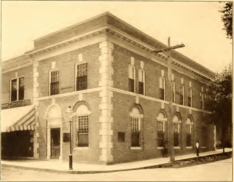
NORWOOD NATIONAL BANK, NORWOOD, MASS. ALLEN & COLLENS, Architects, NEW YORK AND BOSTON.
