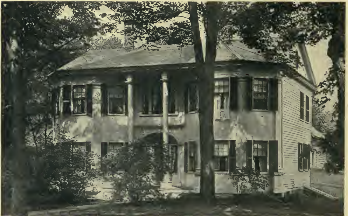
HOUSE AT CASTLETON, VERMONT.
