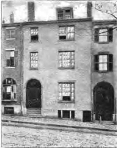
Parkman's Residence, Boston, Mass.
