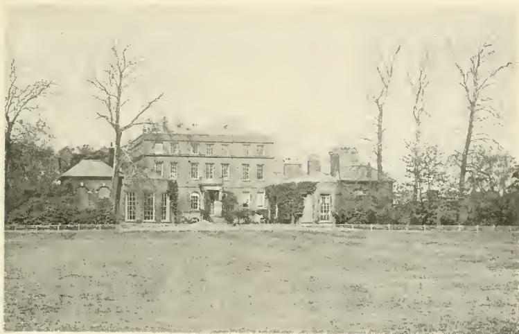
BUSHY HOUSE, EAST FRONT.
