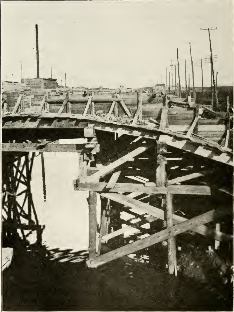
FIG. 1. VIEW OF PILES AND BENTS SHOWING ARRANGEMENT.
