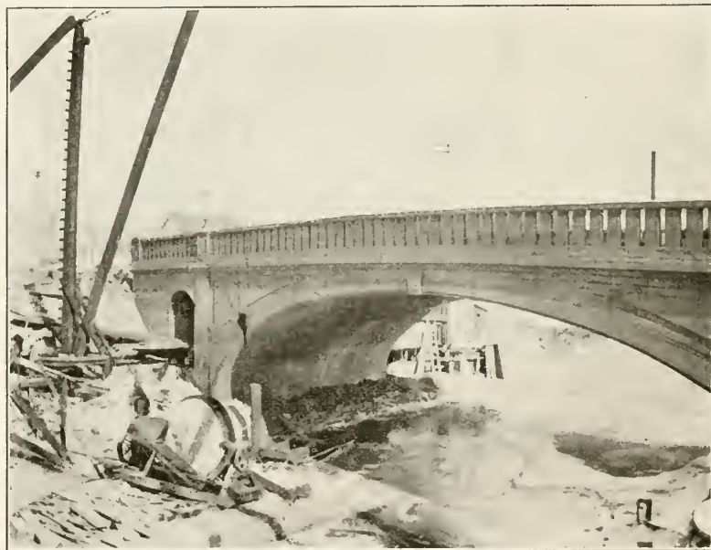
FIG. 7. KEDZIE AVENUE BRIDGE, LOOKING NORTHEAST.
