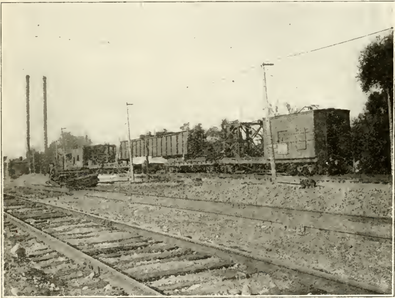
FIG. 17. VIEW OF SLAB ERECTING TRAIN.
