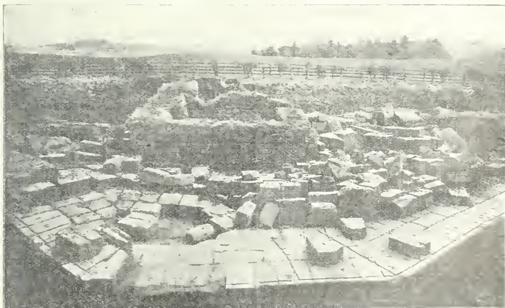
FIG. 3.—Abutment of the Roman bridge at Chesters.
