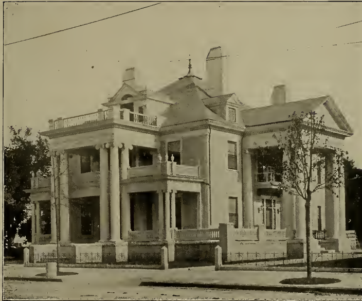
Residence of R. B. Raney, Raleigh, N. C.
