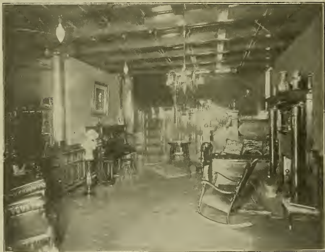
Interior of Staircase Hall, Residence of George L. Lyon.
