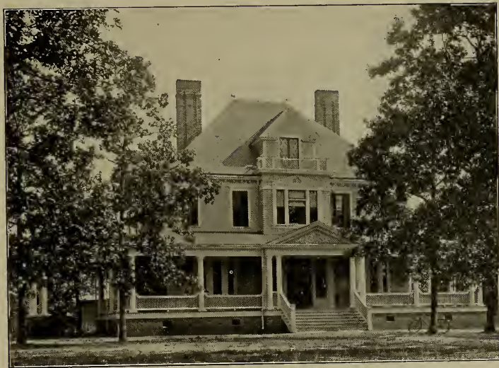
Residence erected at Wake Forest, N. C., for W. C. Powell, of Savannah, Ga.
