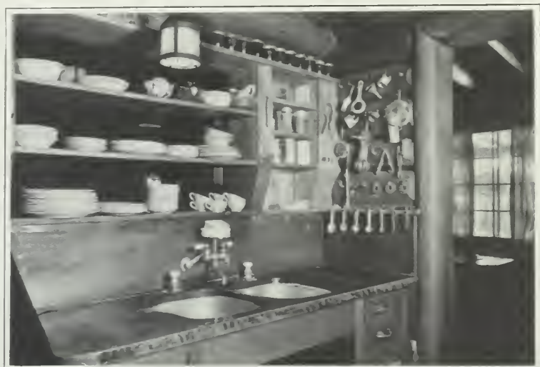
The wide maple-board sink, with mixing faucet and two copper bowls, disposes of the dishpan problem forever. The back of the dish cupboard over the sink drops down in the living room to form the breakfast table
