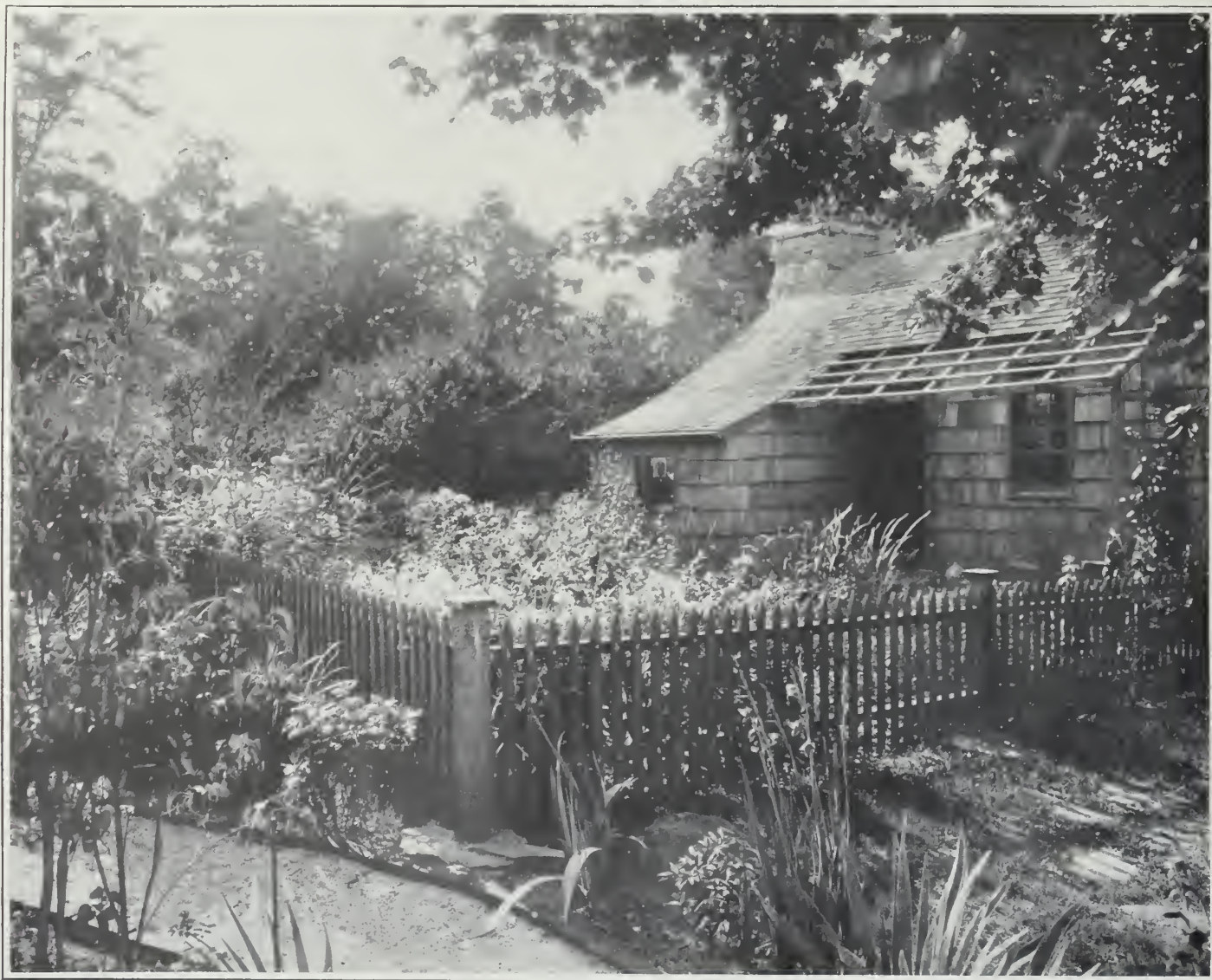
To emphasize the existence of the Little House and its garden as an entirely separate entity from the surrounding grounds, it has its own encircling fence and its own little cottage garden
