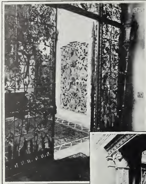
Several dozen birds and animals beautifully wrought give a fantastic charm to the design of a bronze grille which screens the tone opening of an echo organ
