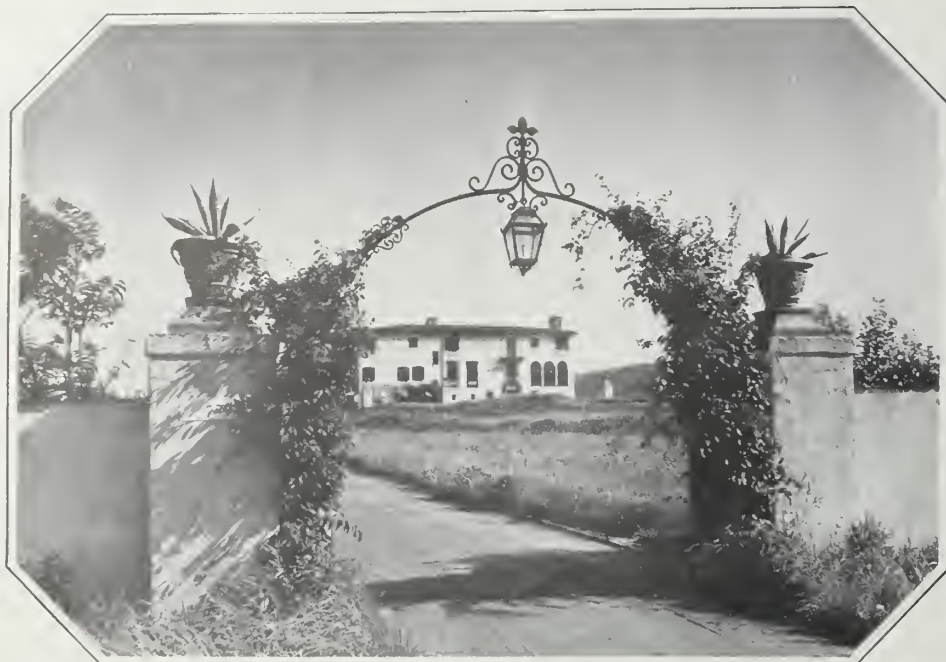
The principal entrance gates. Like the house, the wall and massive gate posts are of stucco
