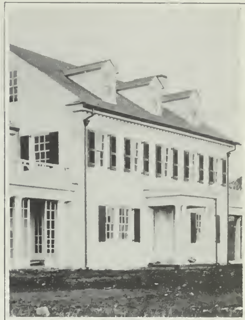
—the same house after the stucco has been applied
