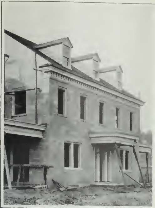
A concrete block house in process of construction, and—
