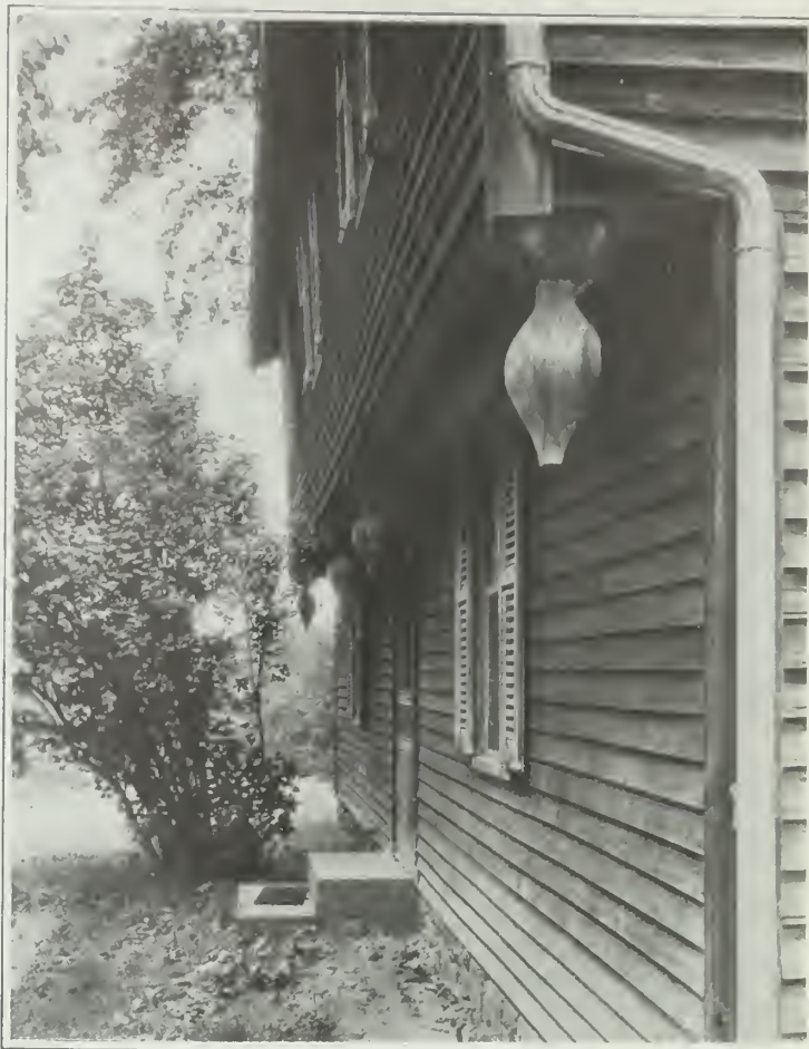
The old Whitman homestead at Farmington, Conn., still taut and trim after its centuries of service. Like most old-time Colonial houses of the North, it is built of white pine
