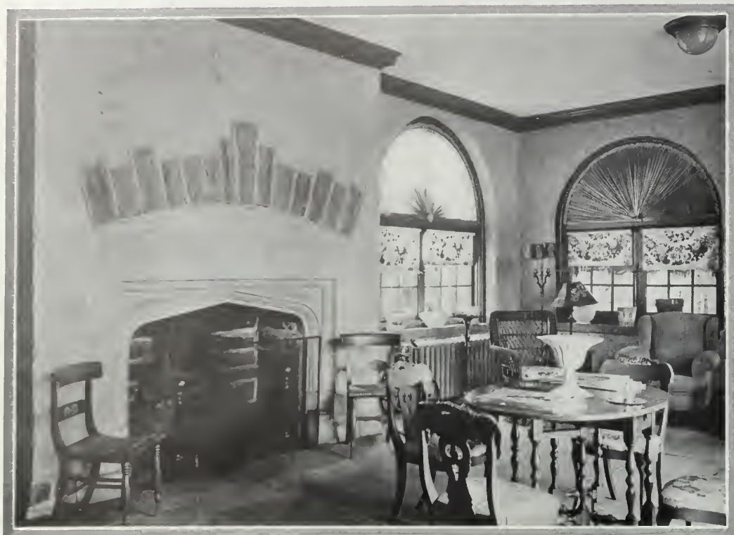
The sun room. The predominating color note here is blue, and the walls are rough stucco. A rather unusual feature is the fireplace lining of large stones, which appear again in the relieving arch of the overmantel
