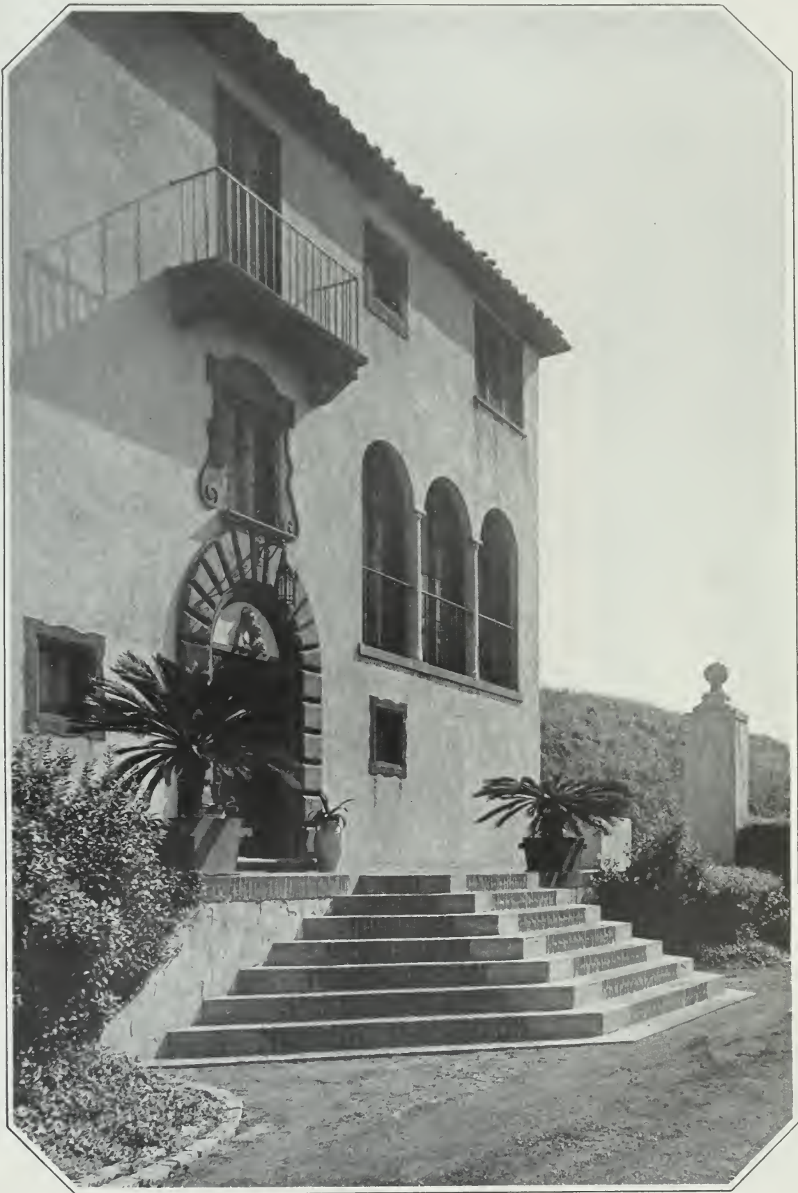
The main entrance to Villa Maria. The architectural detail of the doorway is executed in honed stone, and in the recessed plaster panel above, which is painted a deep blue, is a bas relief of the Virgin and Child. Around the smaller windows the wide raised stucco
