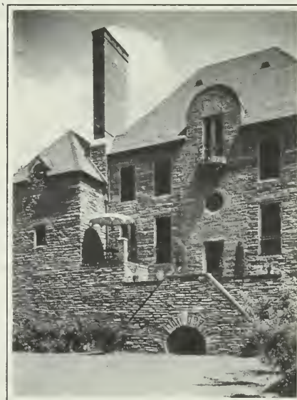
Detail of the front entrance
