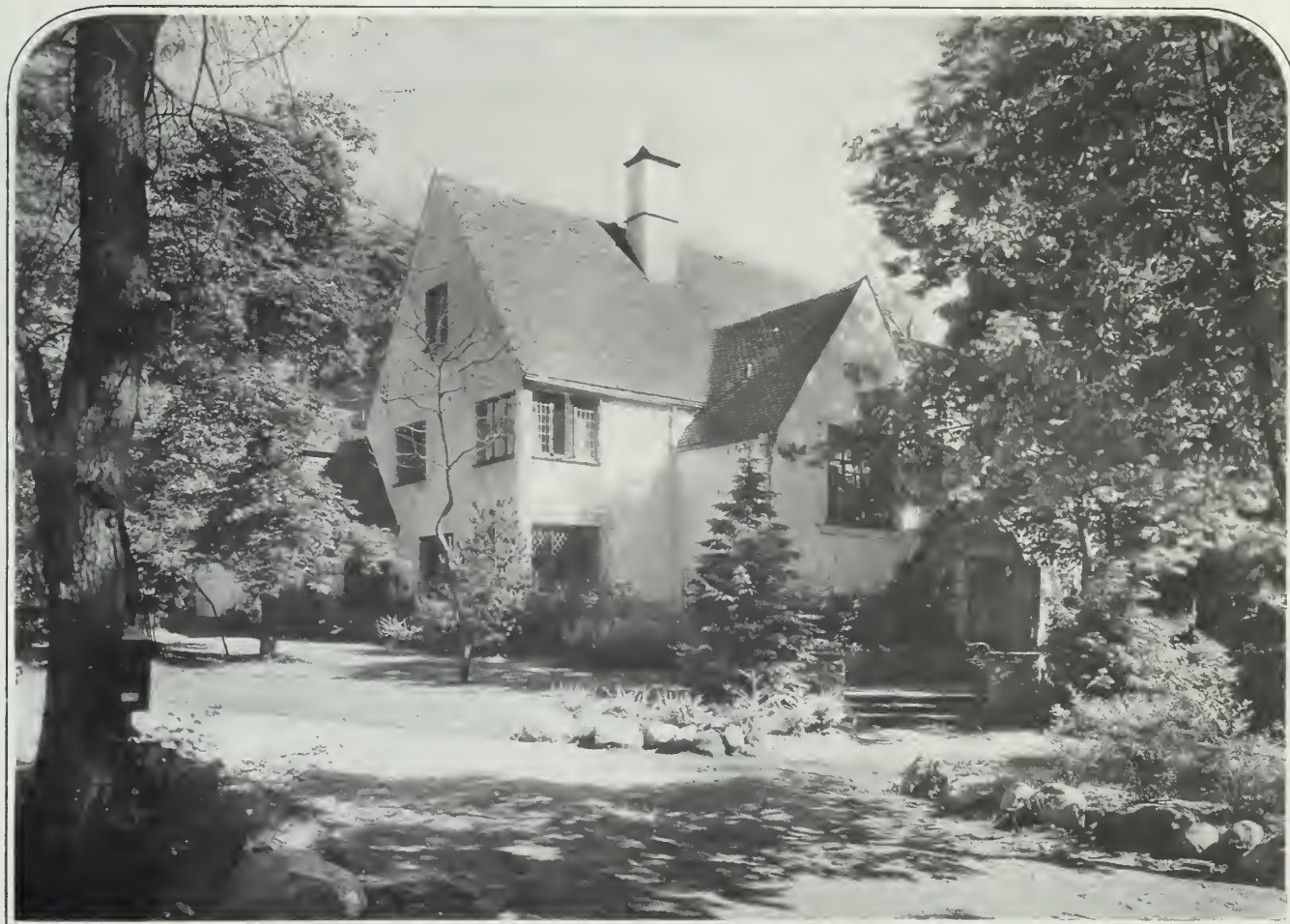
The house is built of hollow tile on a foundation of local stone and the trim is cut limestone, the whole exterior being whitewashed and making an effective foil for the rough slate roof of mottled red and green. As may be gathered from this view, the house is set in a clearing in the woods, and its white walls and mottled roof are in pleasing contrast to the green of the trees
