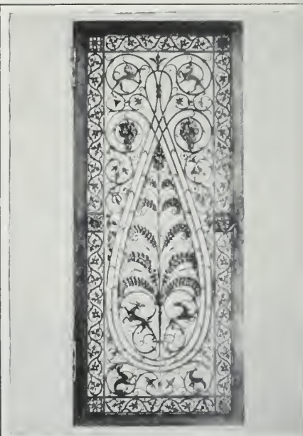
A door whose grille is of forged iron with ornaments of repoussé bronze, shows originality of design, and a daring in motif relation
