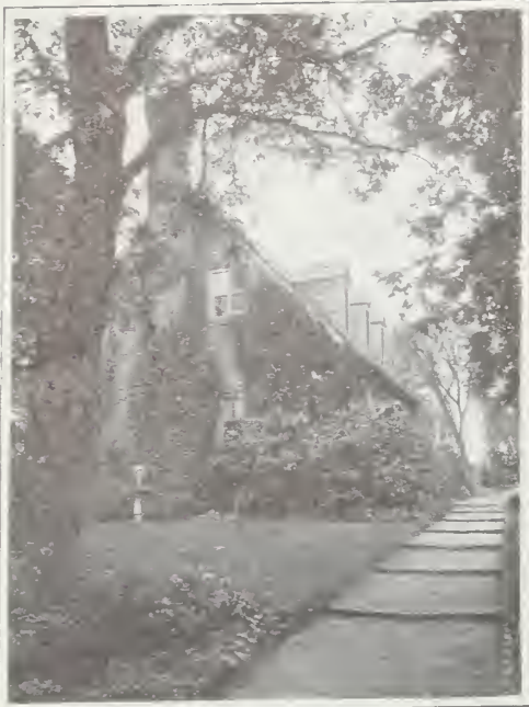
Griffin & Wynkoop, architects of restoration The restored guest cottage at historic York Hall, Yorktown, Va., built in 1693. It has all the character of an English cottage, and is a shining example of the charm that may inhere in the simplest design
