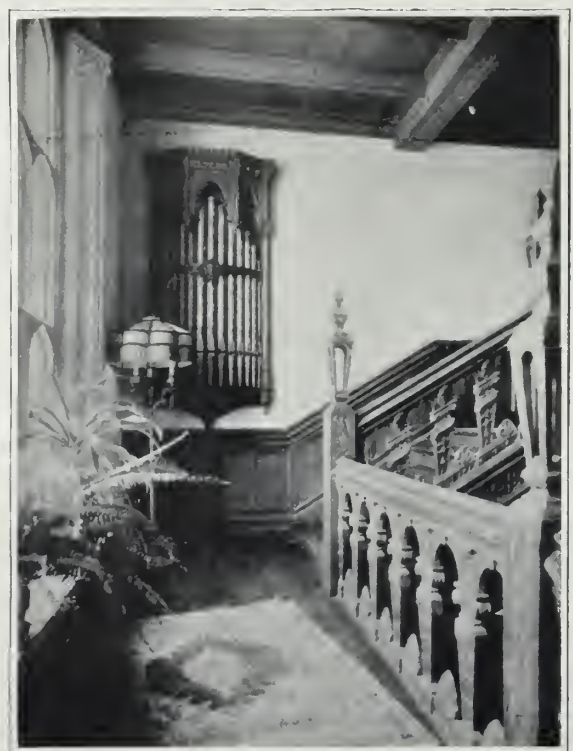
A successful example of the staircase used as the setting for both console and tone outlet. This accomplishes a unity of location that strengthens the decorative harmony. The console is in the space under the stairs (shown at left) and the tone grille on the upper stair wall (at right)
