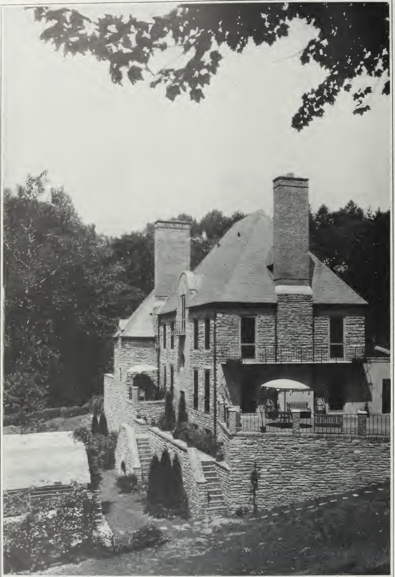
This view of the Illoway house, showing the southeastern terrace, indicates the clever use made of varying levels to give charm and distinction as well as provide outdoor comfort integral with the house. The field stone of which it is built is an admirable medium for retaining walls, steps, etc., and serves to tie house and site into one complete and satisfying whole
