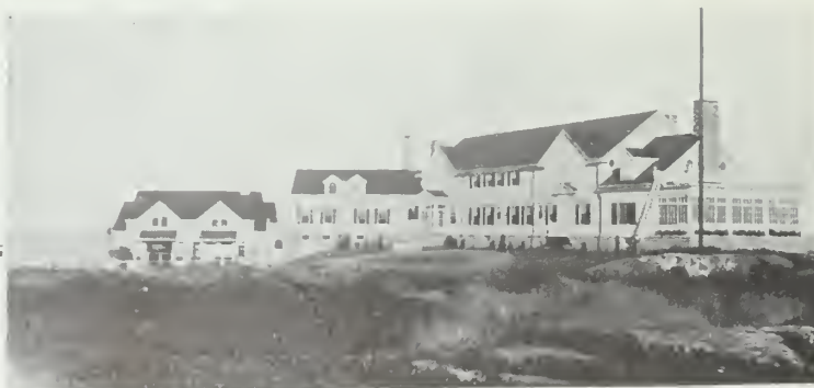
REAR VIEW SHOWING GARAGE, SERVICE WING, ETC.
