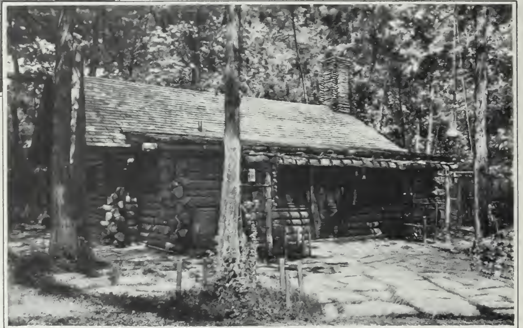
A corner of the cabin (right) with detail of corner construction (above). The tree at the left in both pictures is a hollow white oak log lined with flue tile and connected underground with the machinery pit under the lean-to. It serves as the chimney for the gas-burning heating plant
