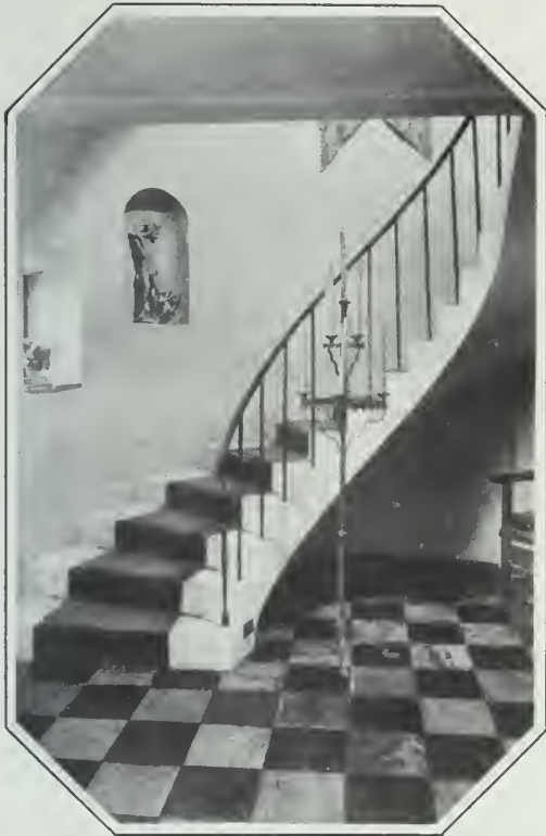
In the stair hall. The gracefully winding staircase that follows the curve of the wall is made of cement painted white, the sharp edges being rounded off to simulate the results of wear
