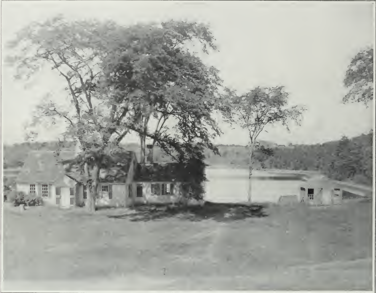
This is one of the Cape cottages such as is described in the accompanying article. A noticeable feature here is the entrance vestibule sometimes found on Cape cottages. This house is rather larger than most and the ell at the right is doubtless quite modern.
