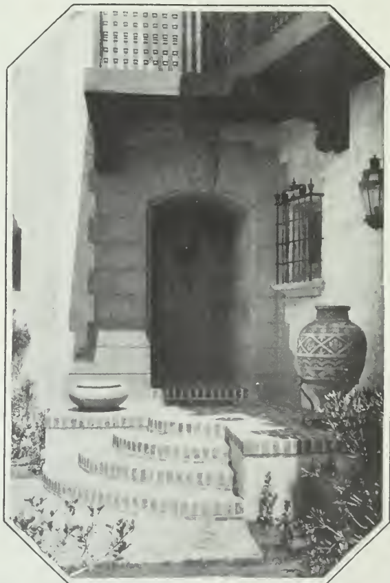
The main entrance is deeply recessed in the wall of the tower, and gives an earnest of the rooms within by its door thickly studded with Moorish nailheads, and an old fourteenth century knocker and grille
