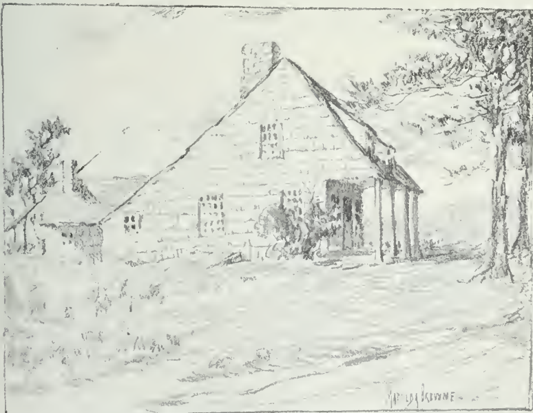
York house at Pleasant Ridge, N. Y., was built by an Englishman of that name, who evidently remembered with affection the dormer windows of old England
