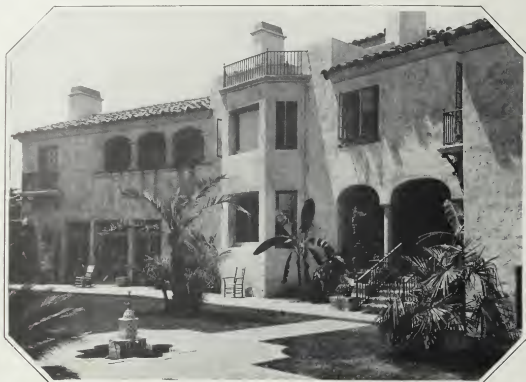
The garden side of the house. The grounds comprise only 170 feet frontage, with a depth of 240 feet, but good use has been made of every inch of space in developing a series of four Old World gardens, each one differing in size, treatment, and details, but all possessing the authentic atmosphere of their ancient prototypes
