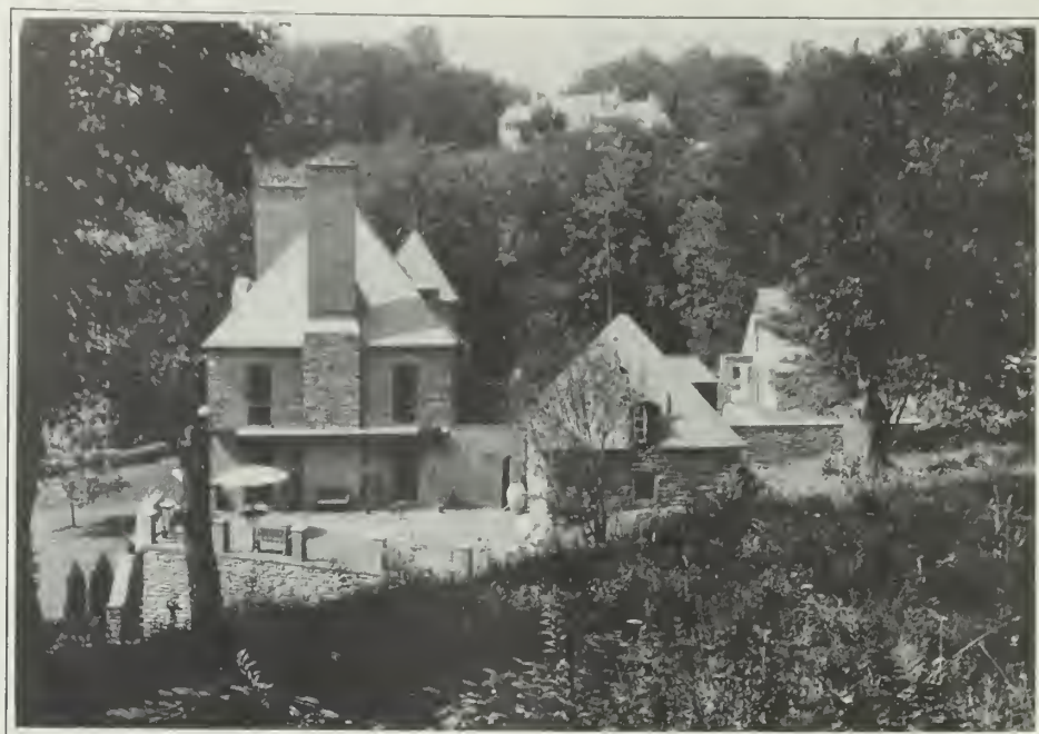
As seen from the east, showing the arrangement of the buildings
