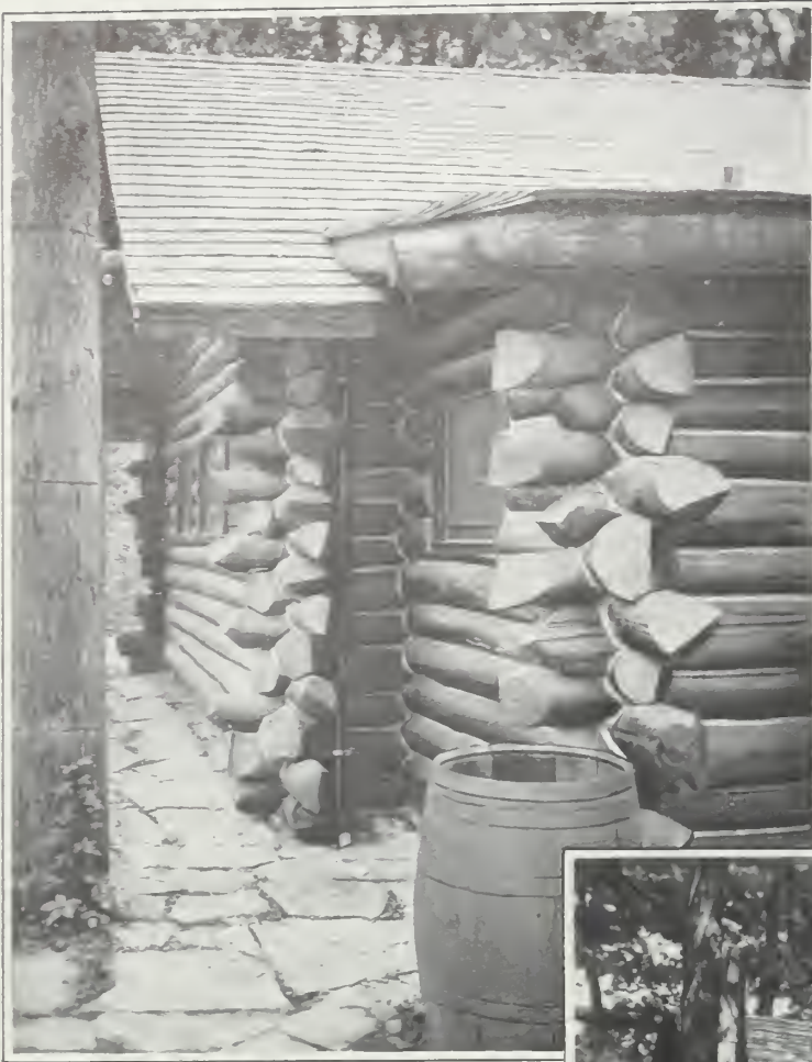
A corner of the cabin (right) with detail of corner construction (above). The tree at the left in both pictures is a hollow white oak log lined with flue tile and connected underground with the machinery pit under the lean-to. It serves as the chimney for the gas-burning heating plant
