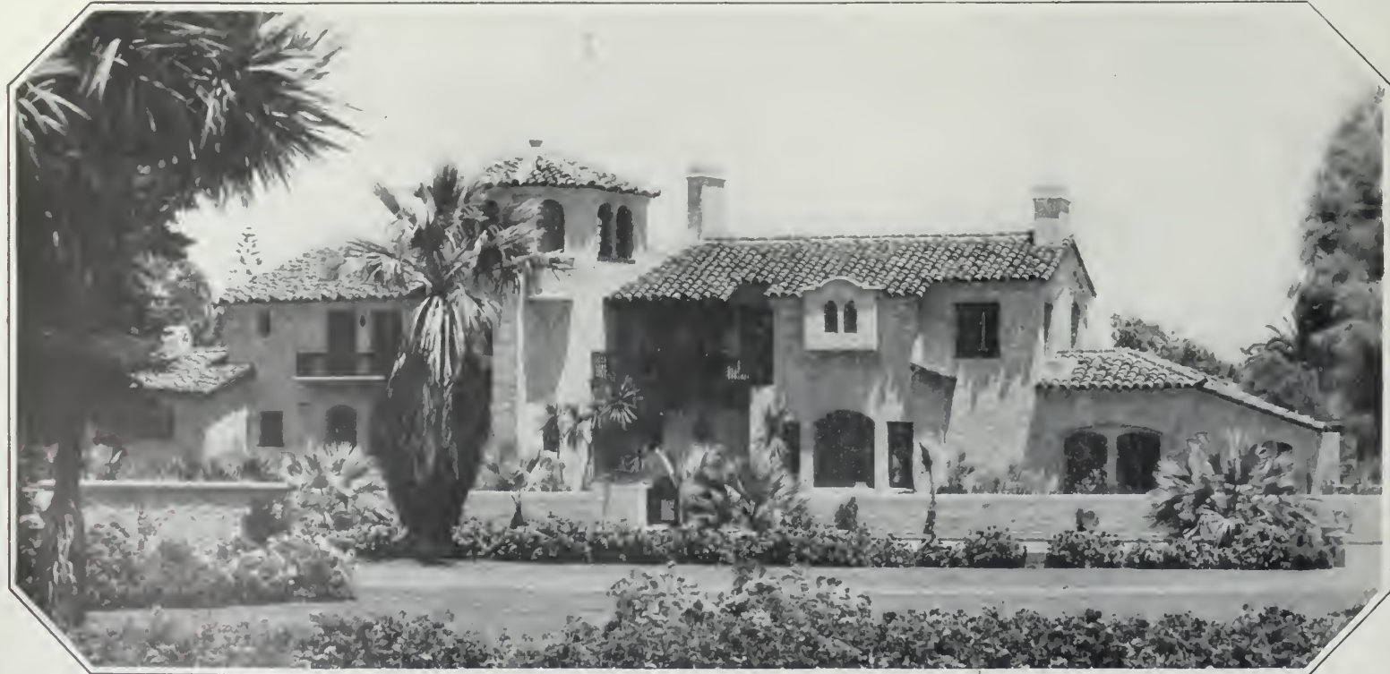
A house at home under tropic skies and with strength to withstand tropic storms, withal it is compounded of romance in line and color and has a picturesque beauty that is notable. The walls are of hollow tile overlaid with dull-toned buff cement put on with free sweeps of the trowel, giving them a texture and interest unknown to the smooth-surfaced wall. The octagonal tower in the center houses a roof garden, from which is an unobstructed view of seashore and mountains, bay and city
