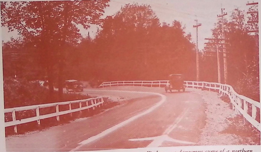
Hand-painted arrow supplemented centerline dividing traffic lanes on dangerous curve of a northern Michigan highway. The nation's first centerline on a rural state highway was laid in 1917 on the Marquette-Negaunee Road (State Trunkline 15) in Marquette County.
