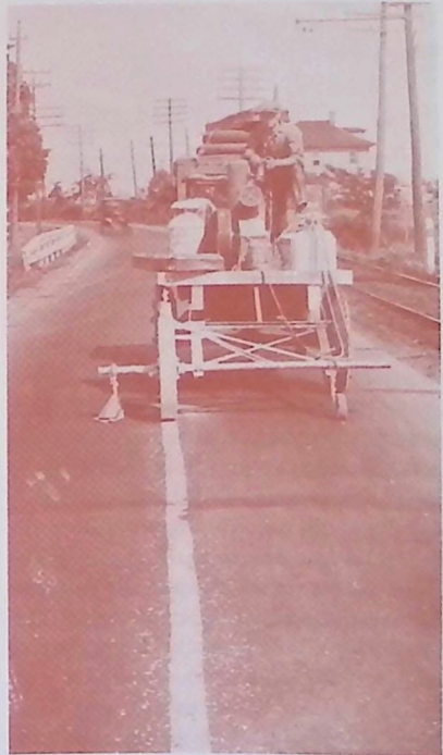
A "Rube Goldberg" type of contraption was used for laying down centerline markings on state highways in the 1920's.
