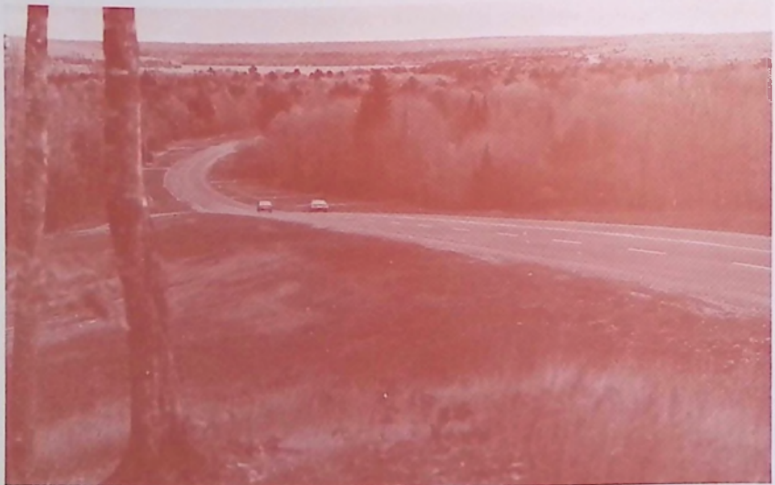
This prize-winning section of M-28 along the shore of Lake Superior typifies Department efforts to upgrade existing highways as well as to build new ones.
