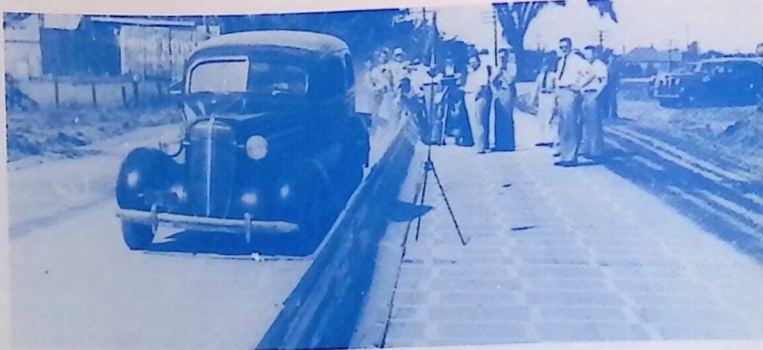
As more and more cars took to the highways in the 1930's, Michigan became a national leader in developing techniques to improve highway safety. Here, safety engineers tested the effectiveness of a guardrail.
