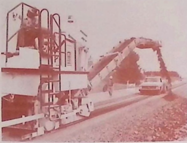
Aging of road surfaces and shortages and increasing costs of oil-based products in the 1970's brought on the recycling of existing pavements.
