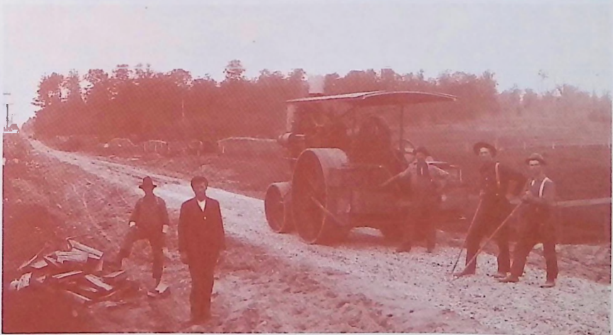
A macadam road, consisting of several layers of crushed stone, was the ultimate in rural highway construction in the early years of the century.
