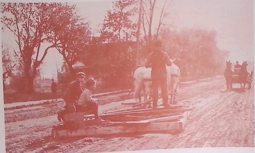
Horses pulling a primitive grader was a standard maintenance technique for Michigan roads in the "Age of Mud."
