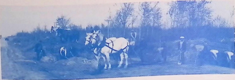
Horses were still important to roadbuilding well into the 1930's. This is a grading and drainage project on M-95 in the western Upper Peninsula in 1935.
