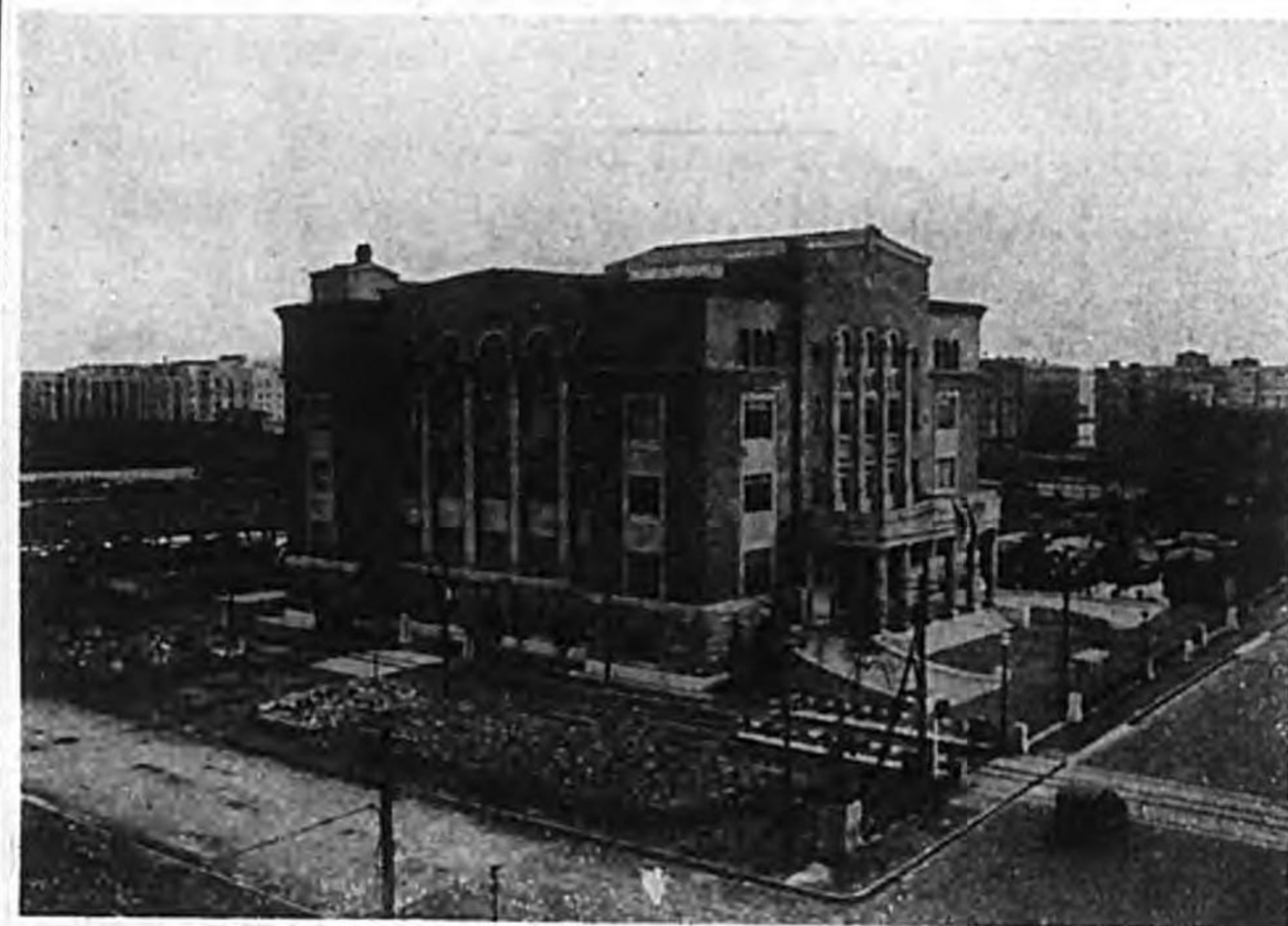
The Kobe Chamber of Commerce and Industry Building, Kyobashi, Kobe
