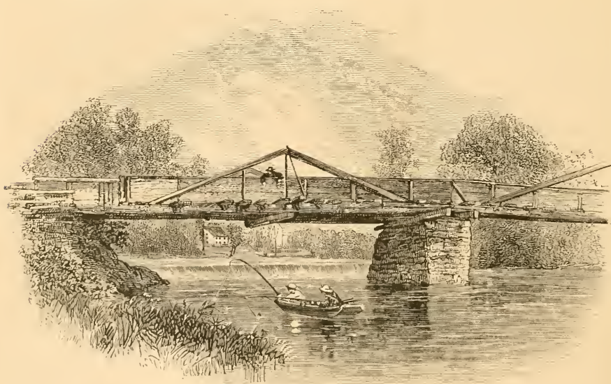
RUSTIC BRIDGE, NORWICH.
