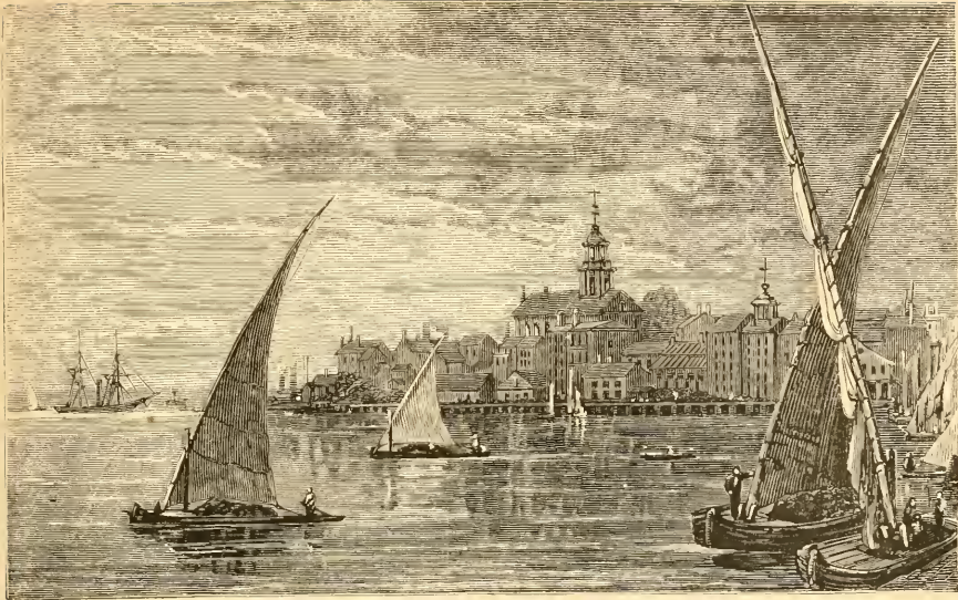
PORTSMOUTH, NEW HAMPSHIRE, FROM KITTERY BRIDGE.
