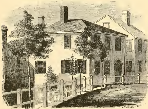
SITE OF THE COMMON HOUSE.
