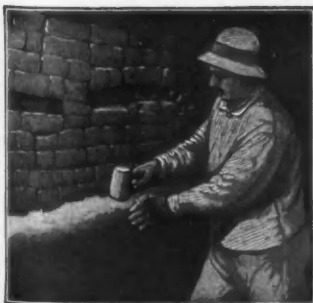
Showing size with which Plibrico is laid in place.
