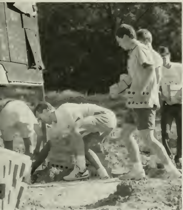
Elon's Habitat chapter starts the foundation on the Delk house. RIGHT: The crew that re-shingled the roof on Kine Street in Burlington.
