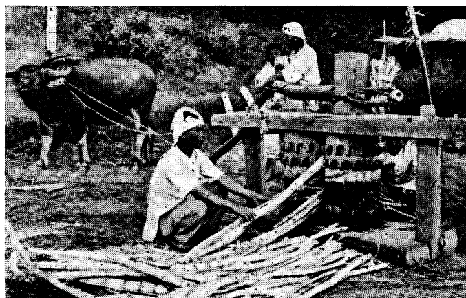
Extracting the Juice of the Sugar Cane
