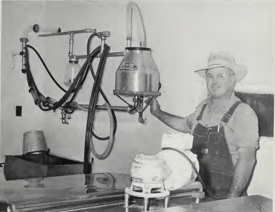
Wilbur Cates, Sayre dairyman, milks 35 cows, says this 440-gallon cooler paid for itself in 3 years by eliminating rejects, and saving on freight and hauling costs.
