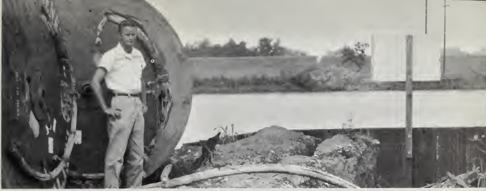
Cable goes under the bayous in some places.
