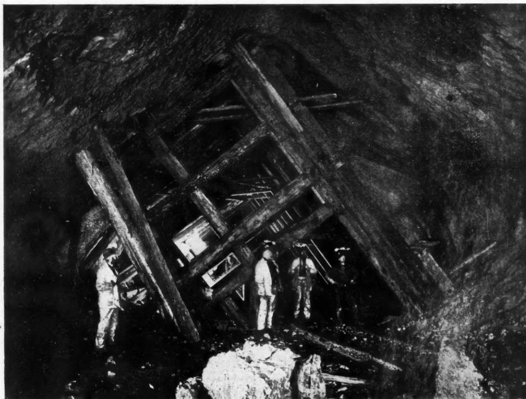
TIMBERING IN THE CALUMET & HECLA MINE, MICHIGAN.
