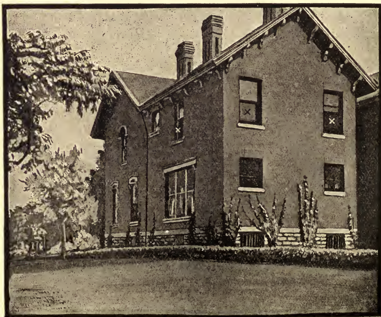
MILBURN MANSION (REAR).
