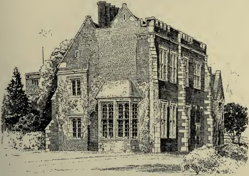
WORMLEIGHTON MANOR-HOUSE, WARWICKSHIRE
