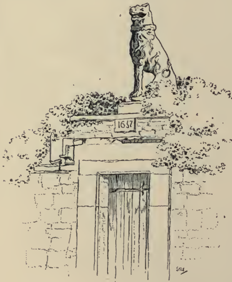
DOORWAY IN GARDEN WALL WINSLEY, WILTSHIRE
