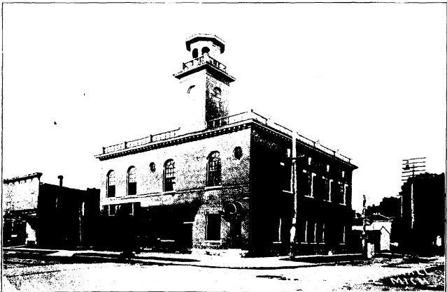
GREENVILLE'S UNIQUE CITY BUILDING.
