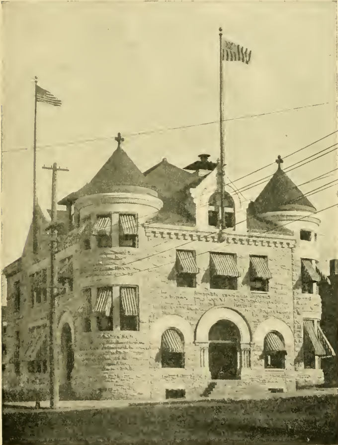
Government building, St. Albans.
