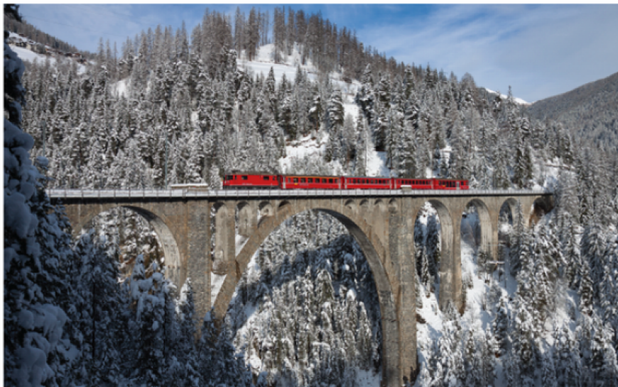
"rhb ge 4-4 ii wiesener viadukt" by Kabelleger, under CC-BY-SA-3.0
