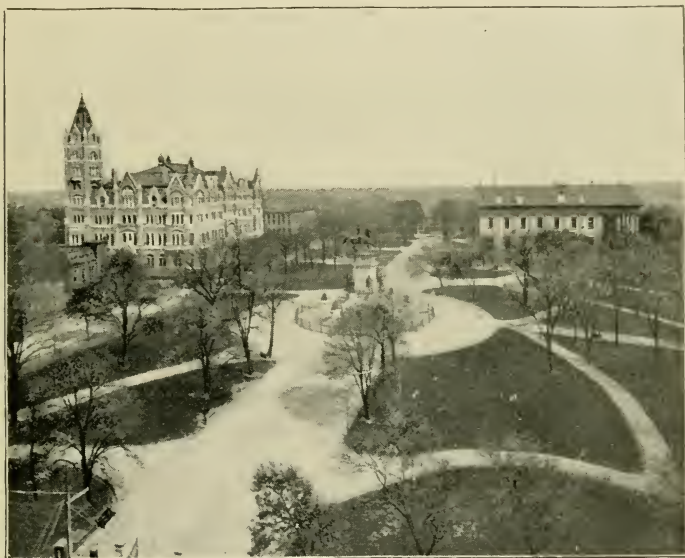
NEW CITY HALL AND CAPITOL SQUARE, RICHMOND.
