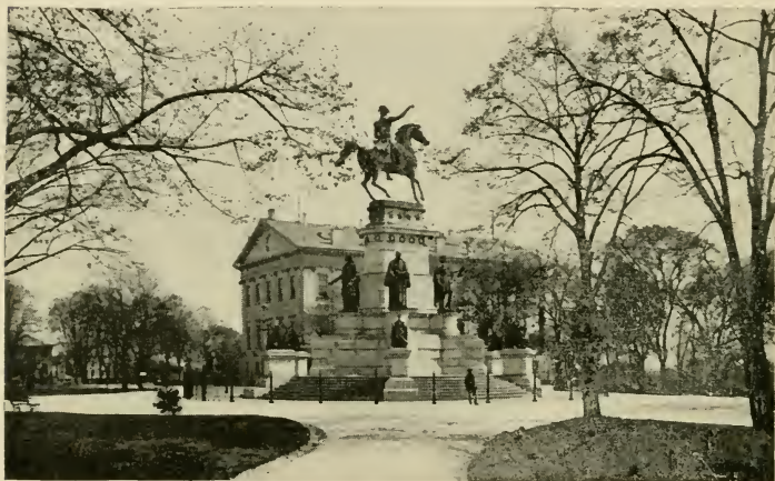
WASHINGTON MONUMENT AND CAPITOL BUILDING, RICHMOND.
