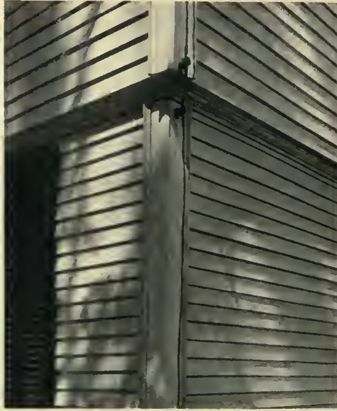
Detail of Corner Boards.
