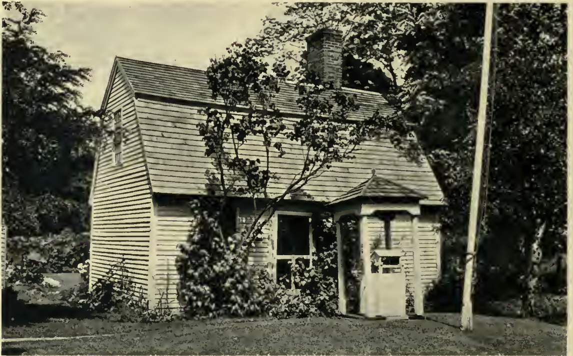
OLD SLAVE QUARTERS OF THE BACON HOUSE, WOODBURY, CONNECTICUT.
