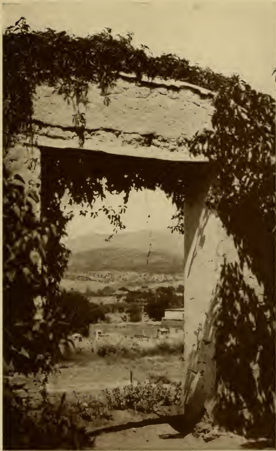
This ancient adobe gateway is among the landmarks of Santa Fe
