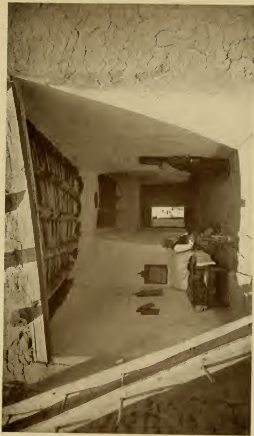
A mud house of the Southwest, being a good example of the massive wall structure, five or six feet thick, employed by the Spanish architects
