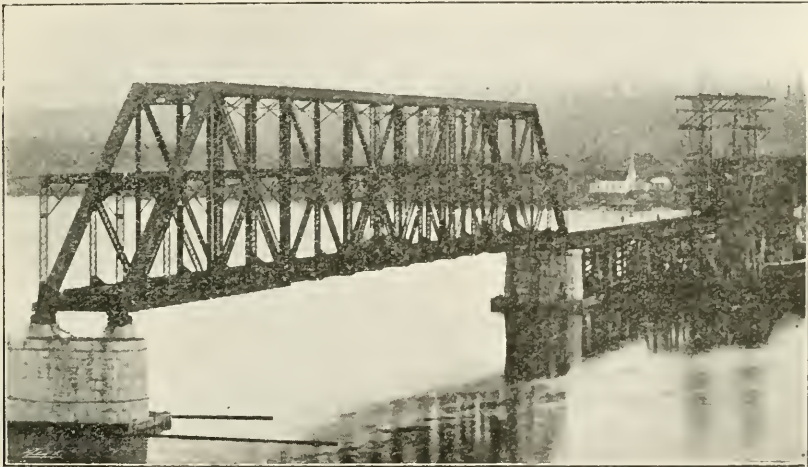
NEW BRIDGE OVER THE FRASER RIVER, NEAR NEW WESTMINSTER, B.C., SHOWING BURNT FORESTS IN DISTANCE.
