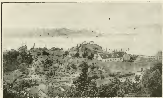
PROTECTION POINT, NANAIMO, SHOWING COAL-SHIPPING WHARVES.
