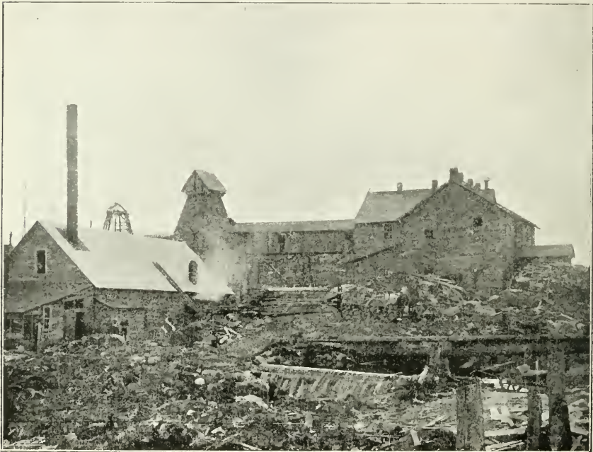
DOMINION NICKEL-COPPER MINE, SUDBURY, ONTARIO—GENERAL VIEW.
