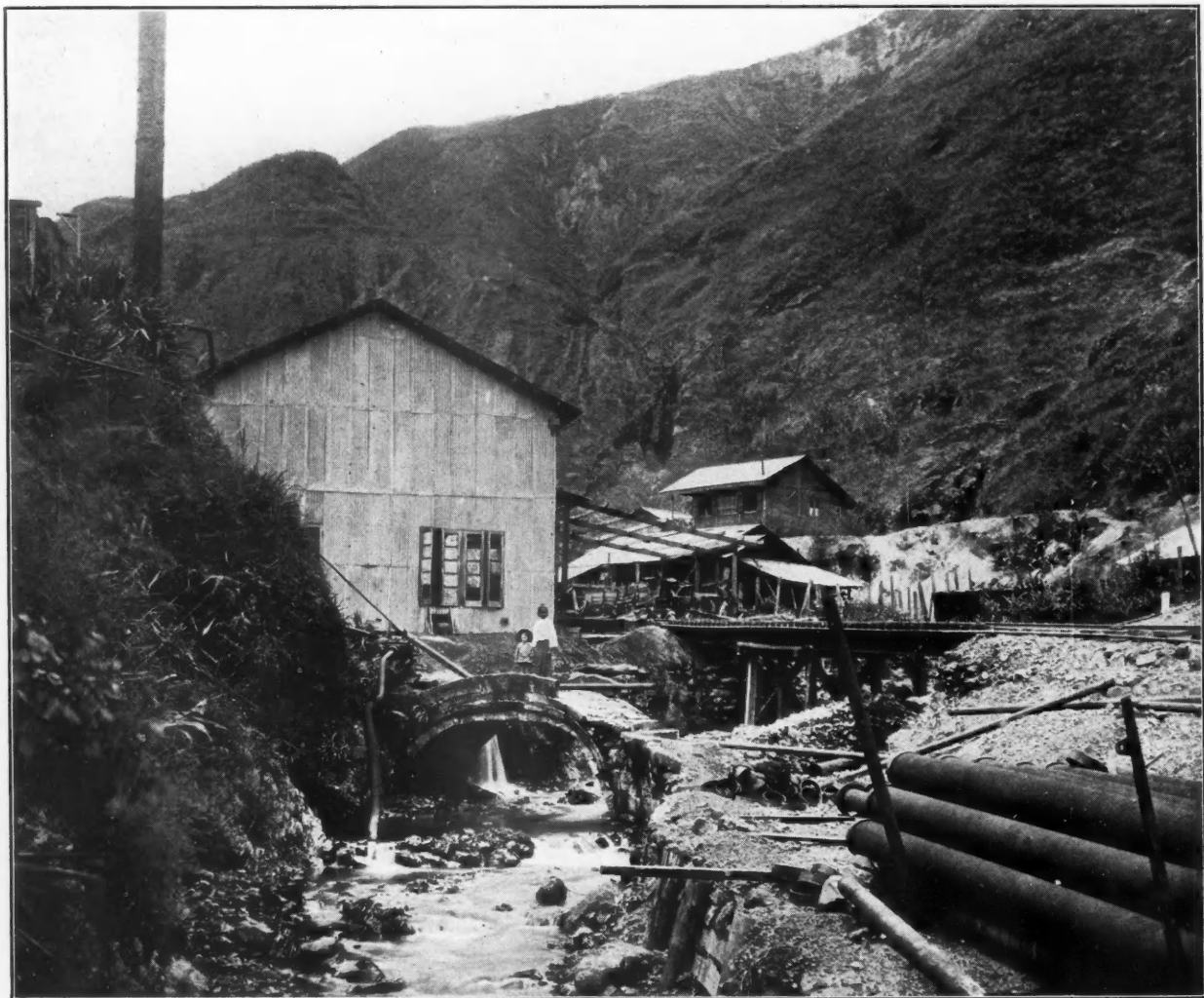
Remains of an old Chinese bridge at Bawdwin
