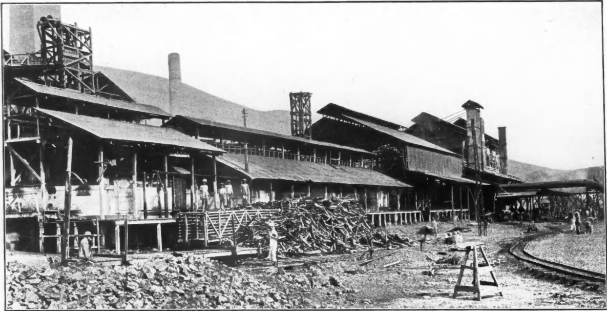
The smelter at Namtu, showing roasters and blast furnaces
