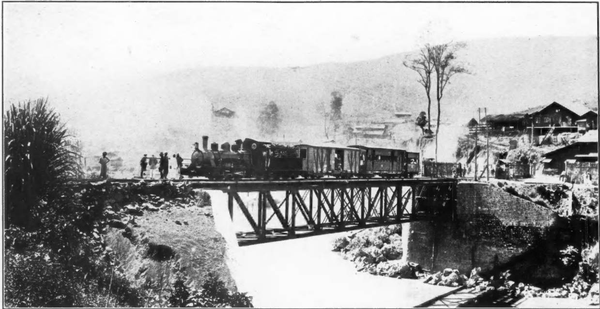
The bridge across the Namtu River, at Namtu
