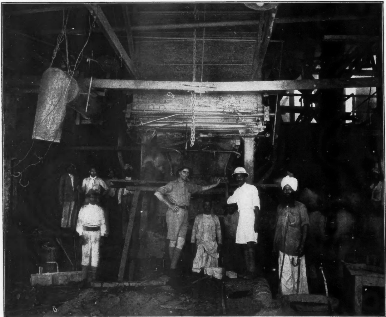
No. 3 blast furnace in course of repair
