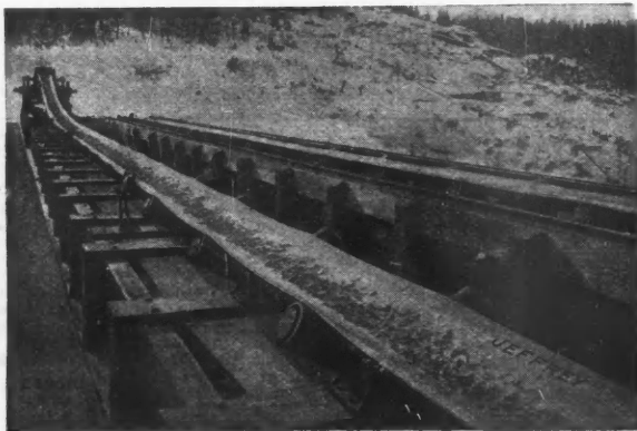
Belt Conveyer with Automatic Tripper distributing to storage bins.
