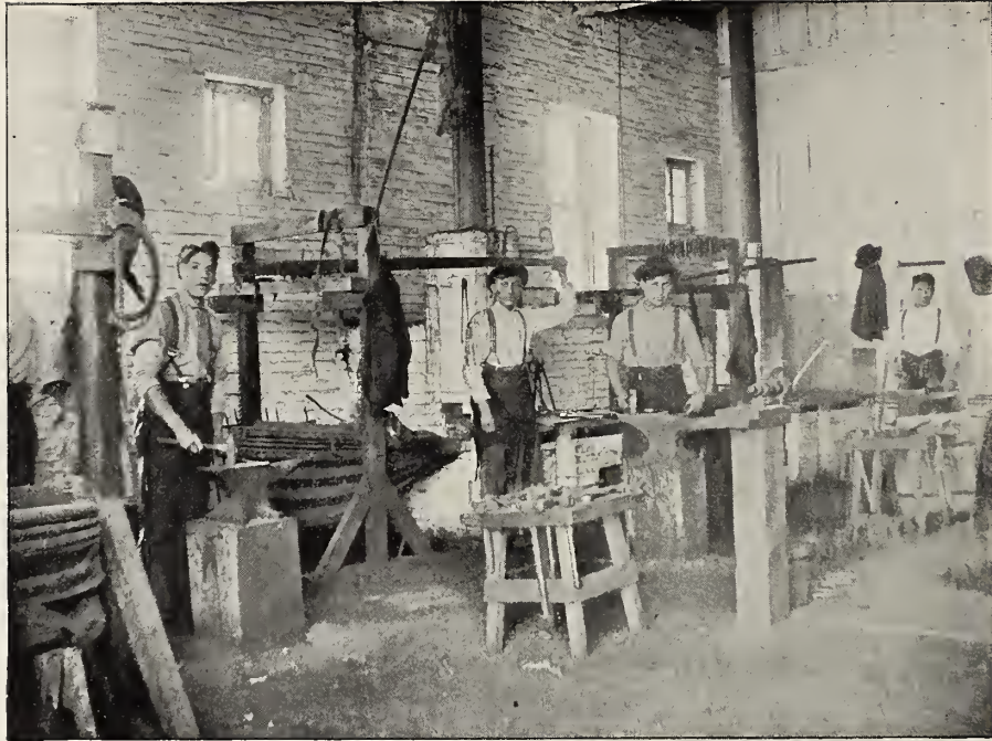
THE BLACKSMITH SHOP INTERIOR
