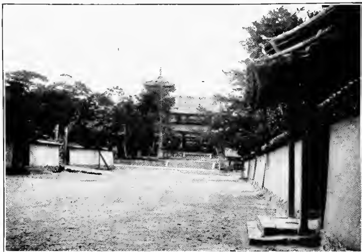
THE OLDEST WOODEN STRUCTURE IN THE WORLD—HORIUJI PAGODA
