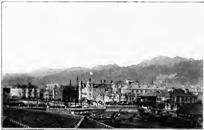
IT WAS NOT KOBE'S FINISHED FRONT THAT GAVE IT AN APPEARANCE OF SUCCESS, BUT ITS UNFINISHED STATE
