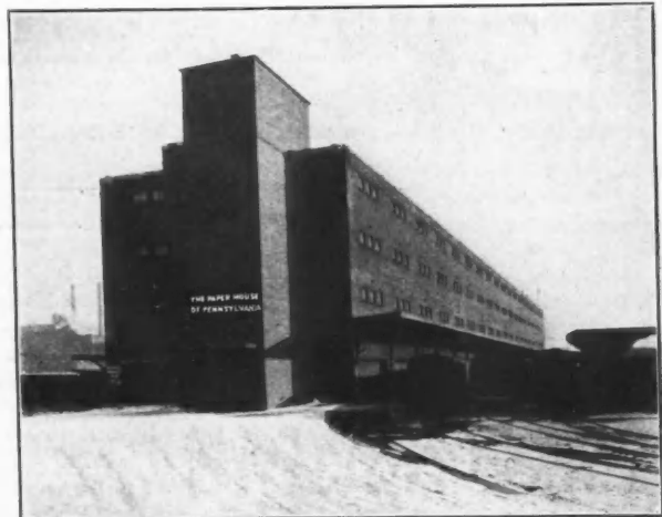
EXTERIOR OF WAREHOUSE, FRONT AND FEDERAL STREETS, SHOWING RAILROAD FACILITIES
