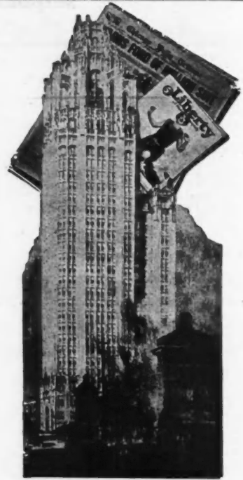
The Chicago Tribune's new Tower Building under construction in Chicago.
