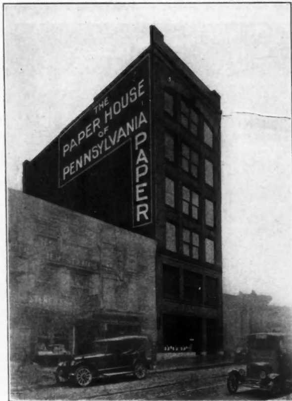
MAIN OFFICE, 28-30 NORTH 6TH STREET, PHILADELPHIA.
