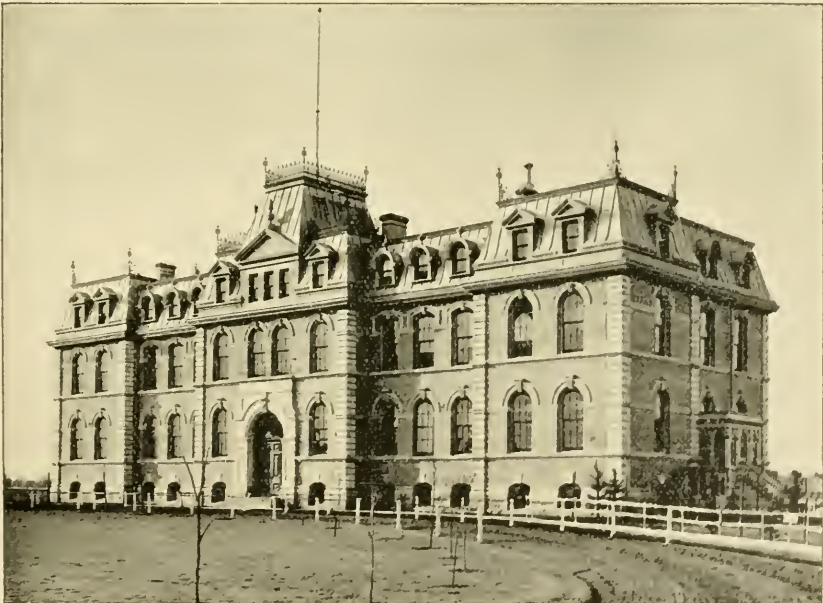
19. MANITOBA GOVERNMENT BUILDING, WINNIPEG, 1897.
